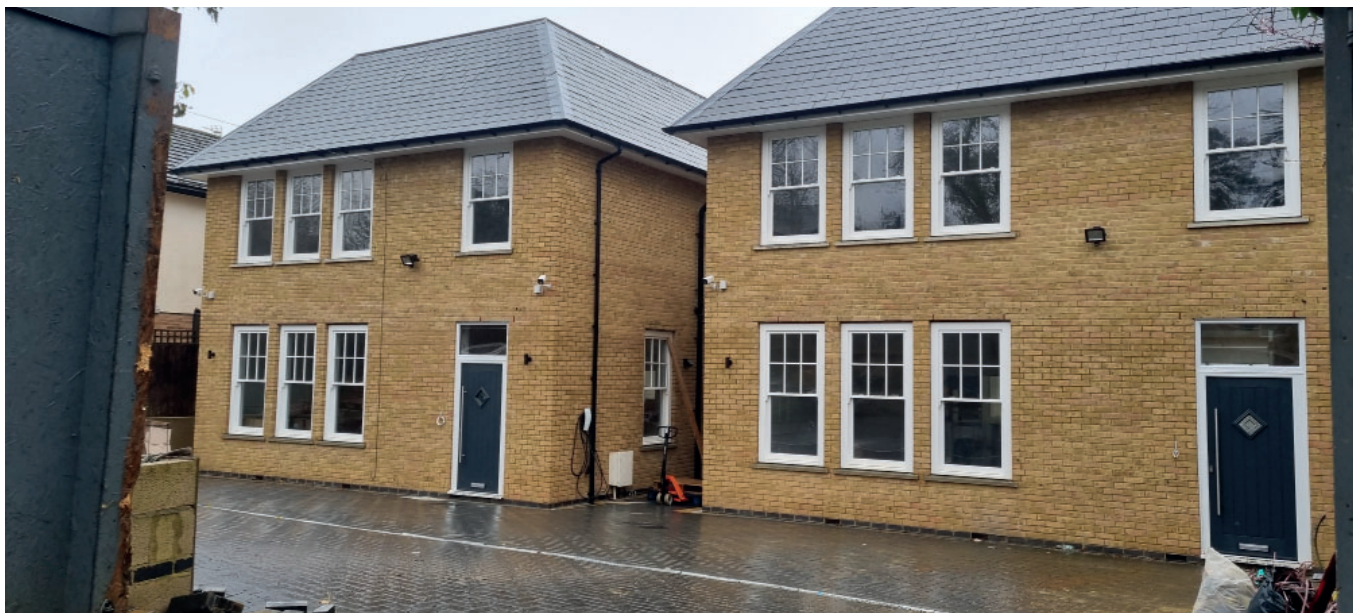
Fig. 17. Replacement dwellings at No. 15 Oaklands Road, north side
