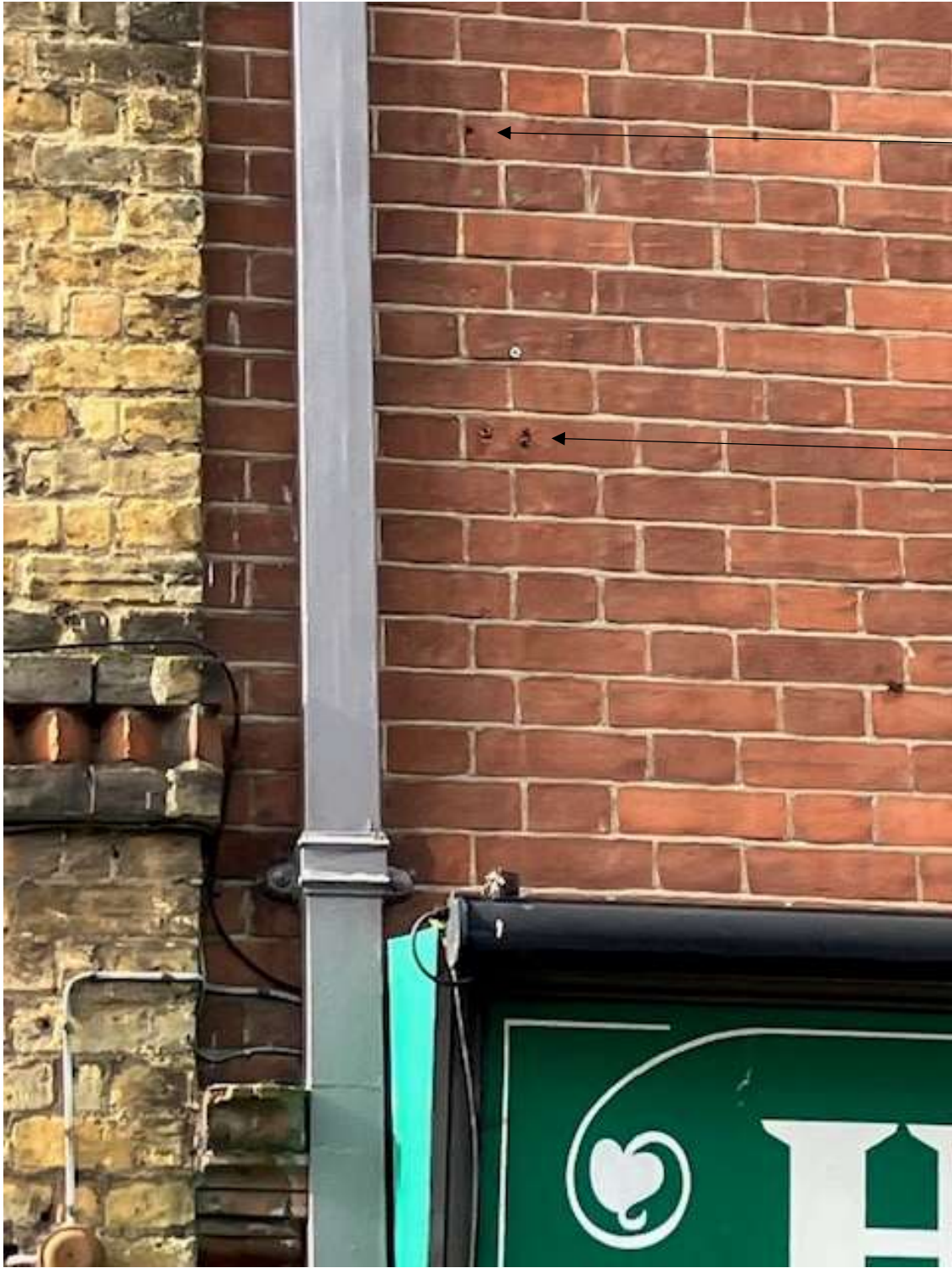
Fig 8: Picture showing numerous screw holes indicating that different hanging signs have been present in the past.
