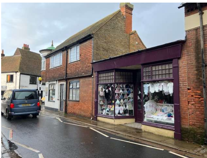
Fig 6: The buildings directly opposite are of a mixed and different style.
