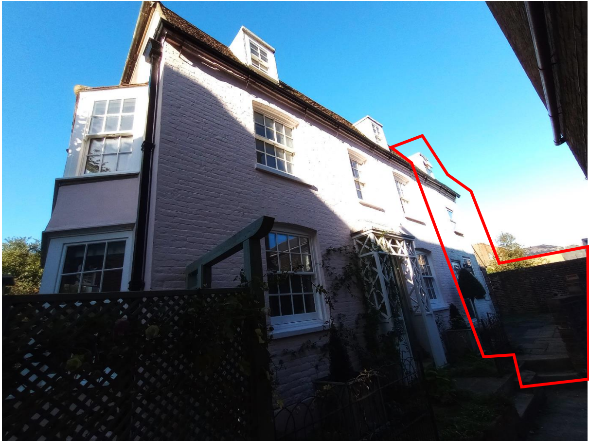
Figure 2 Prospect House is a period property that isn't listed. Access is along a narrow alley behind restaurant refuse storage bins
