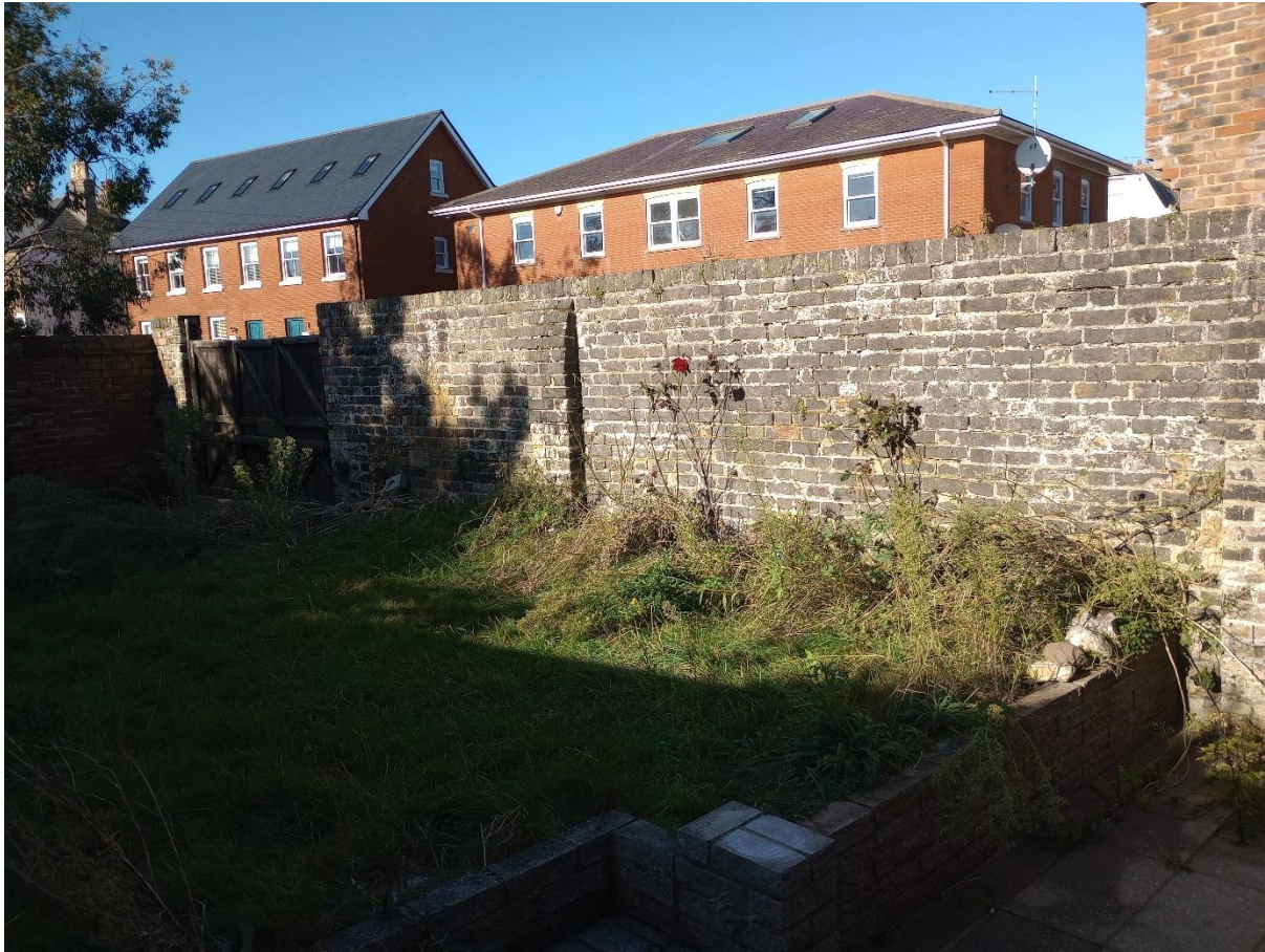
Figure 7 Garden boundary wall with three storey residential apartments beyond.
