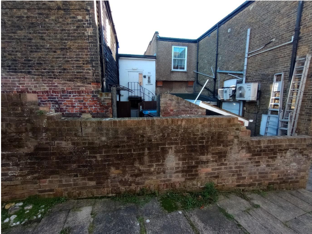
Figure 4 Beyond the boundary brick wall is the back of house bin storage of high street restaurants.
