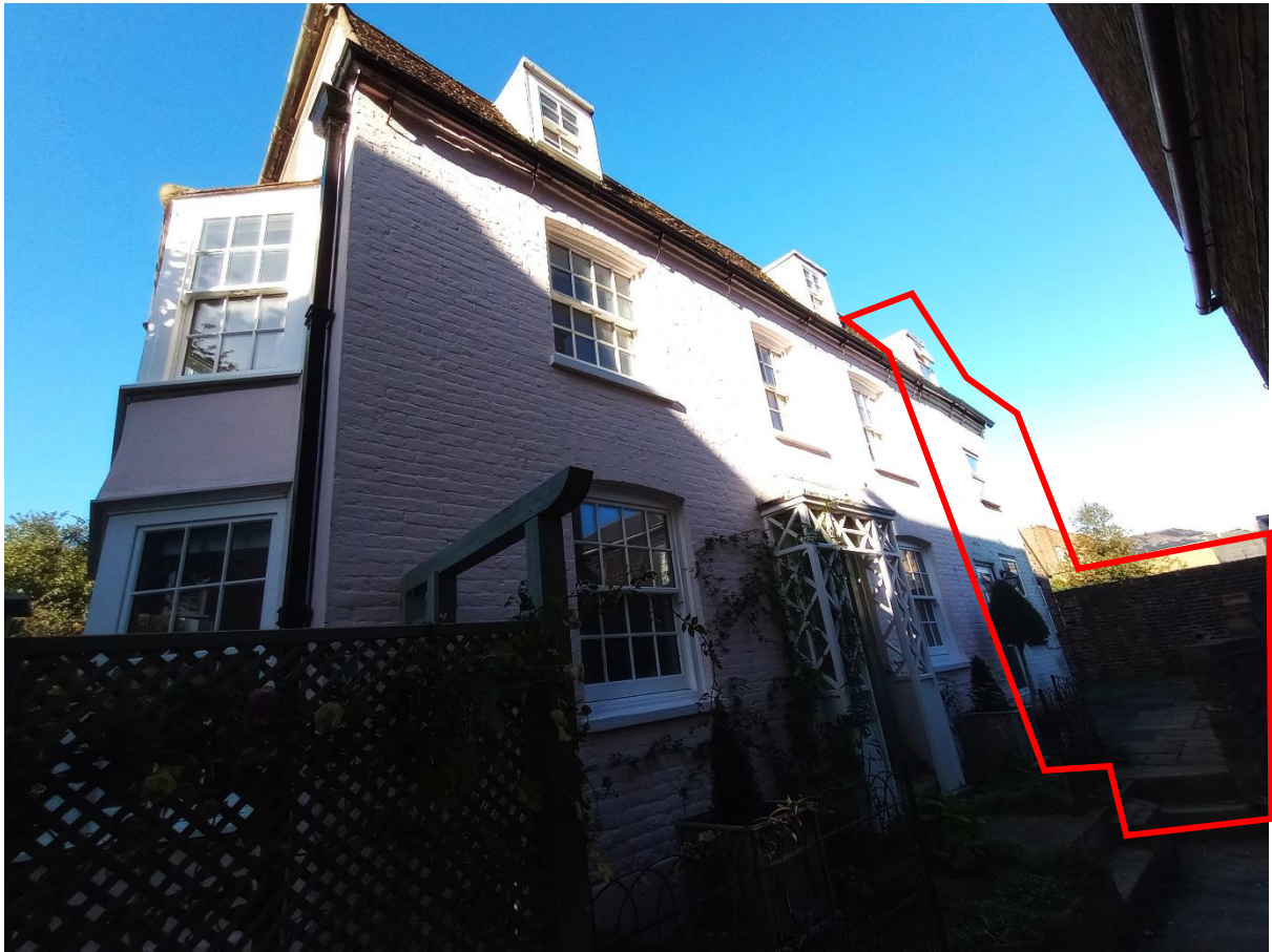
Figure 3 Prospect House is a period property that isn't listed. Access is along a narrow alley behind restaurant refuse storage bins
