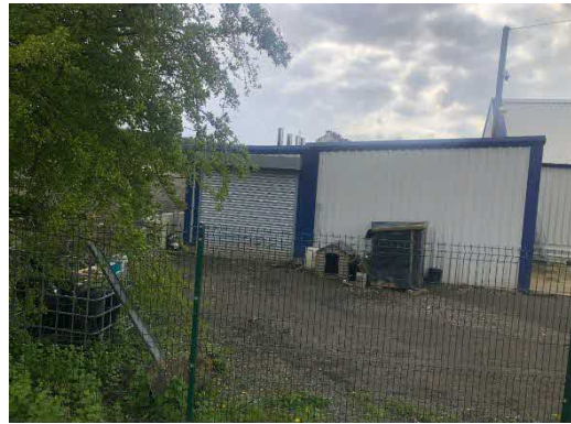
Northern Elevation from Eldon Road
