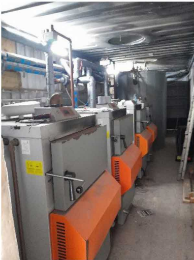
Self contained boiler room in steel container showing Solar Bayer wood burning boilers.
