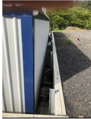
Retaining wall at east elevation.
