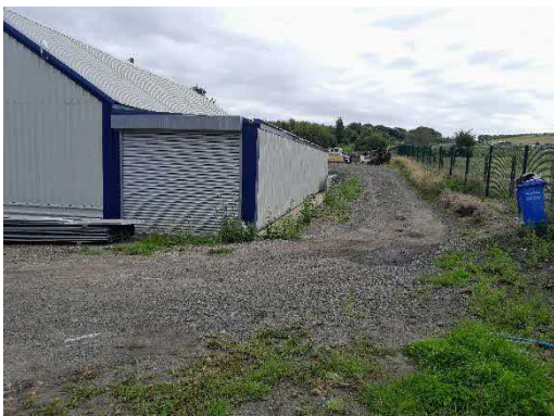
Southern Elevation looking East
