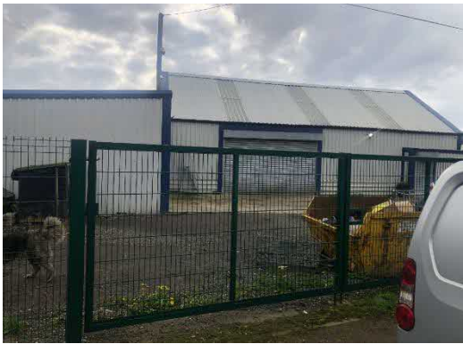
Northern Elevation from Eldon Road
