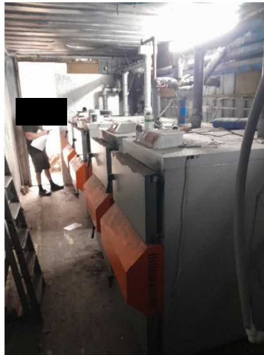
Self contained boiler room in steel container showing Solar Bayer wood burning boilers.
