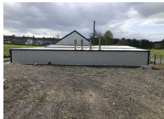
East Elevation showing flues.
