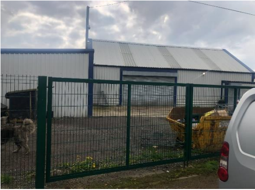
Northern Elevation from Eldon Road
