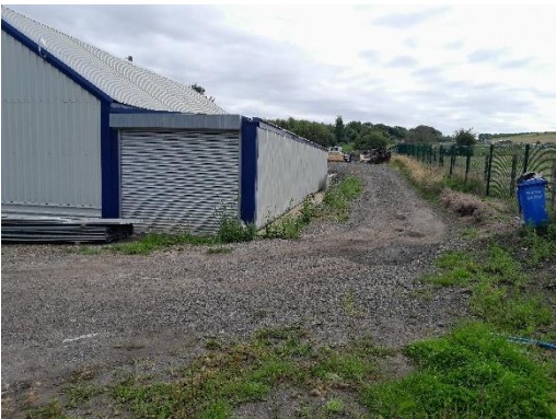
Southern Elevation looking East
