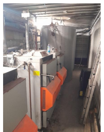
Self contained boiler room in steel container showing Solar Bayer wood burning boilers.
