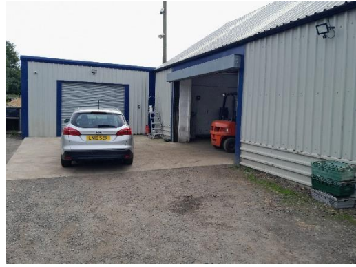
Store after infill cladding and roller door installed
