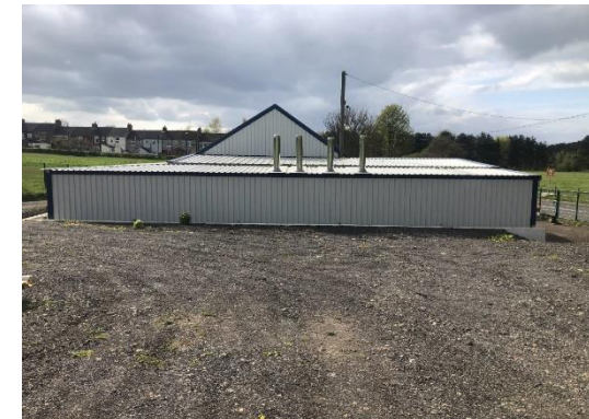
East Elevation showing flues.
