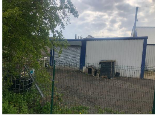
Northern Elevation from Eldon Road
