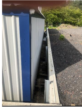
Retaining wall at east elevation.
