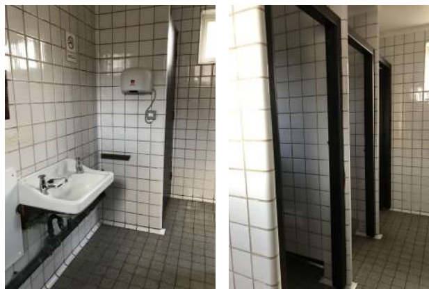
Photos 04 and 05: Public Toilet Block interior
