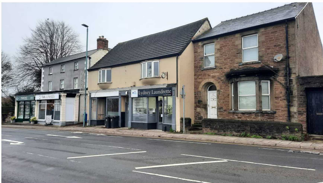
Photograph 1. Existing shop front facing onto the High Street showing both shop fronts with central door providing access to flat over. Shop frontage to remain unaltered during the new scope of improvements. Note render work to high level and concrete slates to roof.
