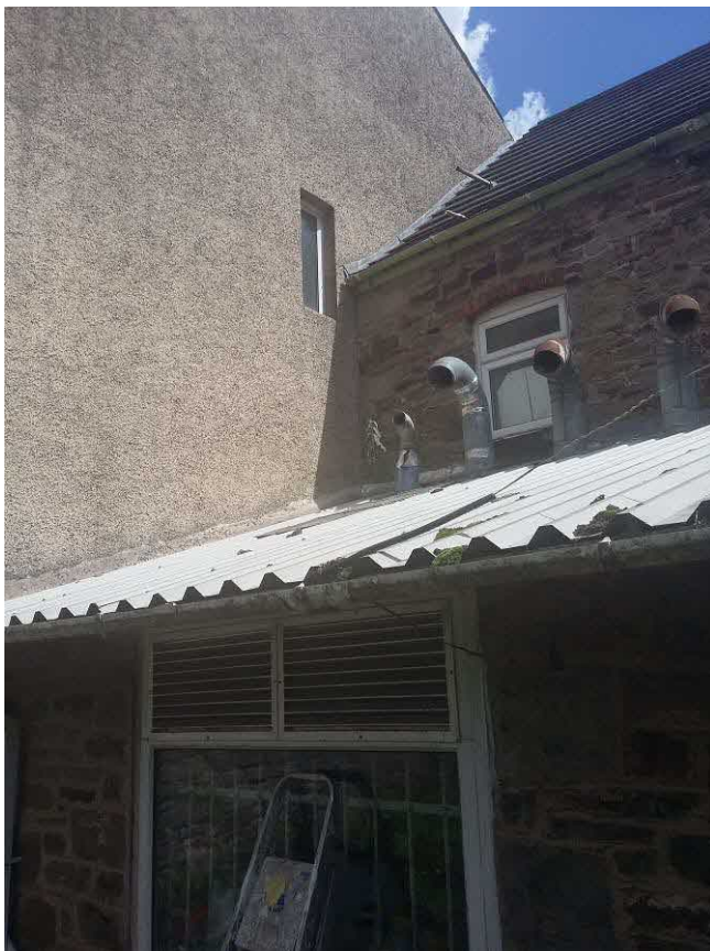
Photograph 5. Existing rear elevation. Notice window to neighbour and rough cast finish to neighbour plus lower eaves height to rear
