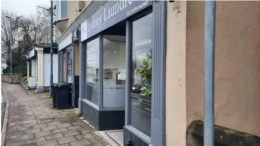
Photograph 2. Front elevation showing older style shop front and render work
