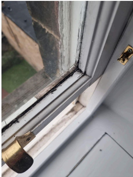
Broken putty and rotting woodwork to new windows.
