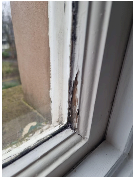
Rotting pulley stile and internal woodwork.
