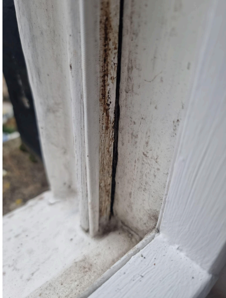
Rotting parting beads and baton rods
