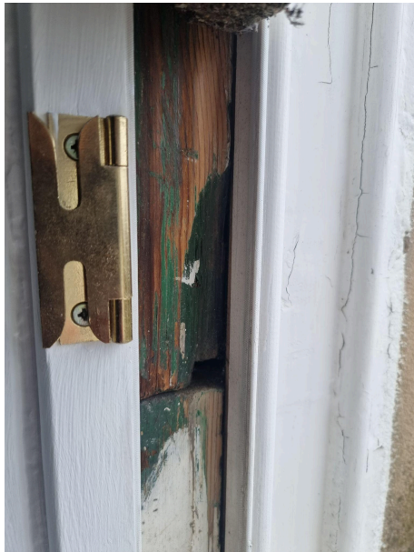
Rotting pulley stile and internal woodwork.
