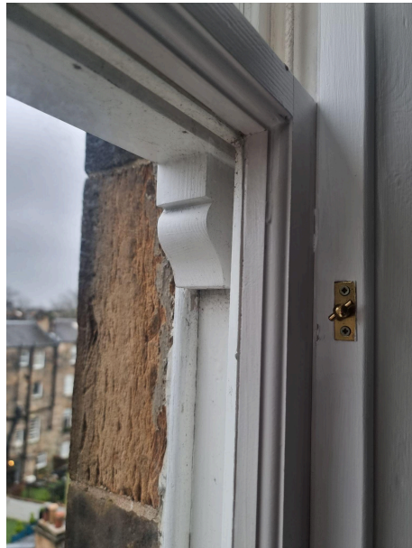
Modern horn details and internal molds showing that the windows have been replaced.
