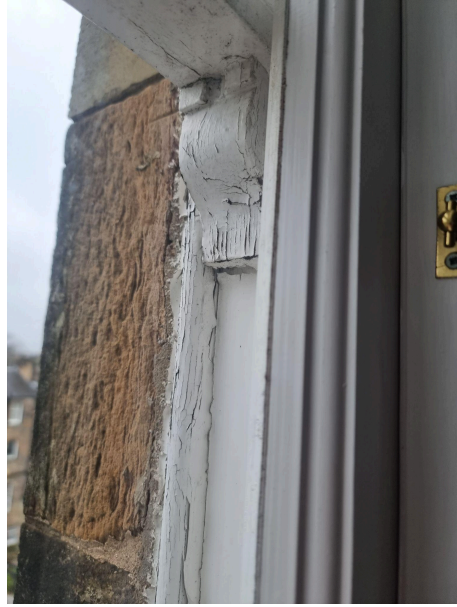
Older style horn details which are deteriorating and rotting.
