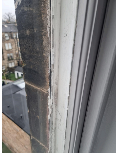
Deteriorating and rotting woodwork to external casement.
