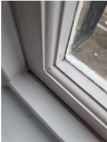
Modern horn details and internal molds showing that the windows have been replaced.
