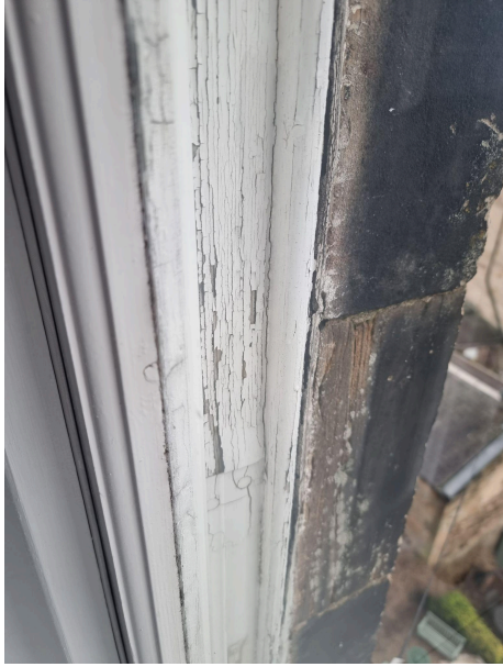
Deteriorating and rotting woodwork to external casement.
