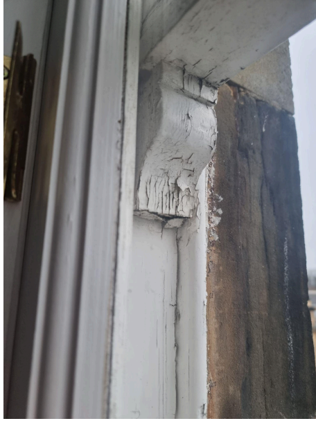
Older style horn details which are deteriorating and rotting.
