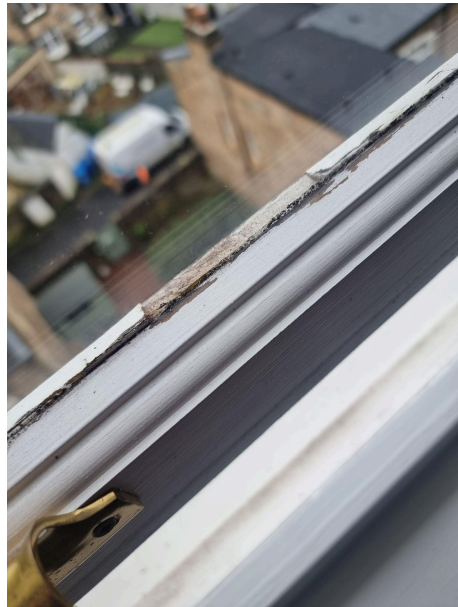
Broken putty and rotting woodwork to new windows.
