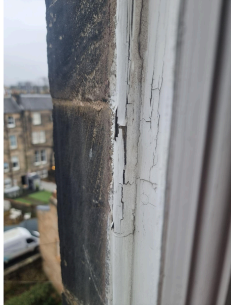
Rotting parting beads and baton rods
