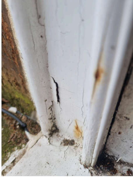
Casement and external woodwork of bottom sash has bubbling and peeling paint to the woodwork which is allowing water to penetrate the soft pine woodwork and escalating the deterioration. Woodwork is damp and showing signs of rot underneath.
