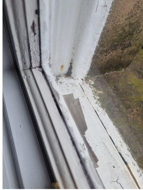
Casement and external woodwork of bottom sash has bubbling and peeling paint to the woodwork which is allowing water to penetrate the soft pine woodwork and escalating the deterioration. Woodwork is damp and showing signs of rot underneath.
