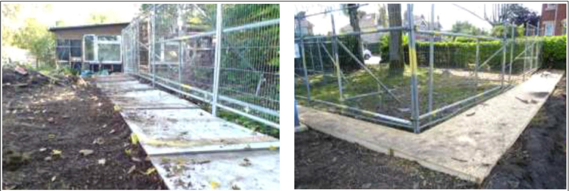
Examples of temporary ground protection suitable for pedestrian movements only - heavy-duty plywood sheets pinned into position (left) and plywood sheets fixed to a timber framework (right)
