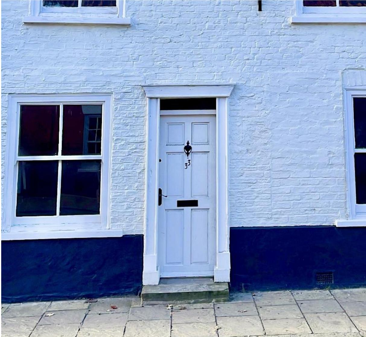
The proposed new front door is a Colonial 6 Panel External Meranti Door and Frame that is sized at 1981x762mm (very slightly larger than the current 1950x760mm door) in size. The overall frame would be an almost like-for-like replacement to what we currently have, with an overall height of 2062mm and 844mm width.
