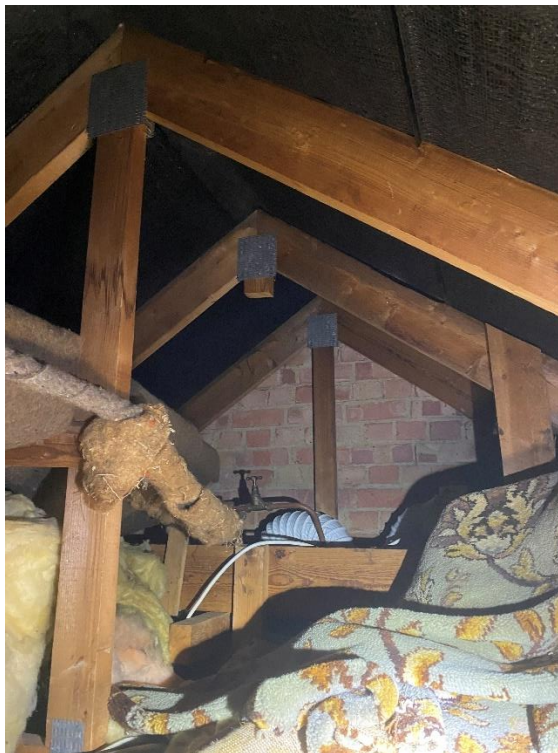
Photograph 3: Internal view of loftspace
