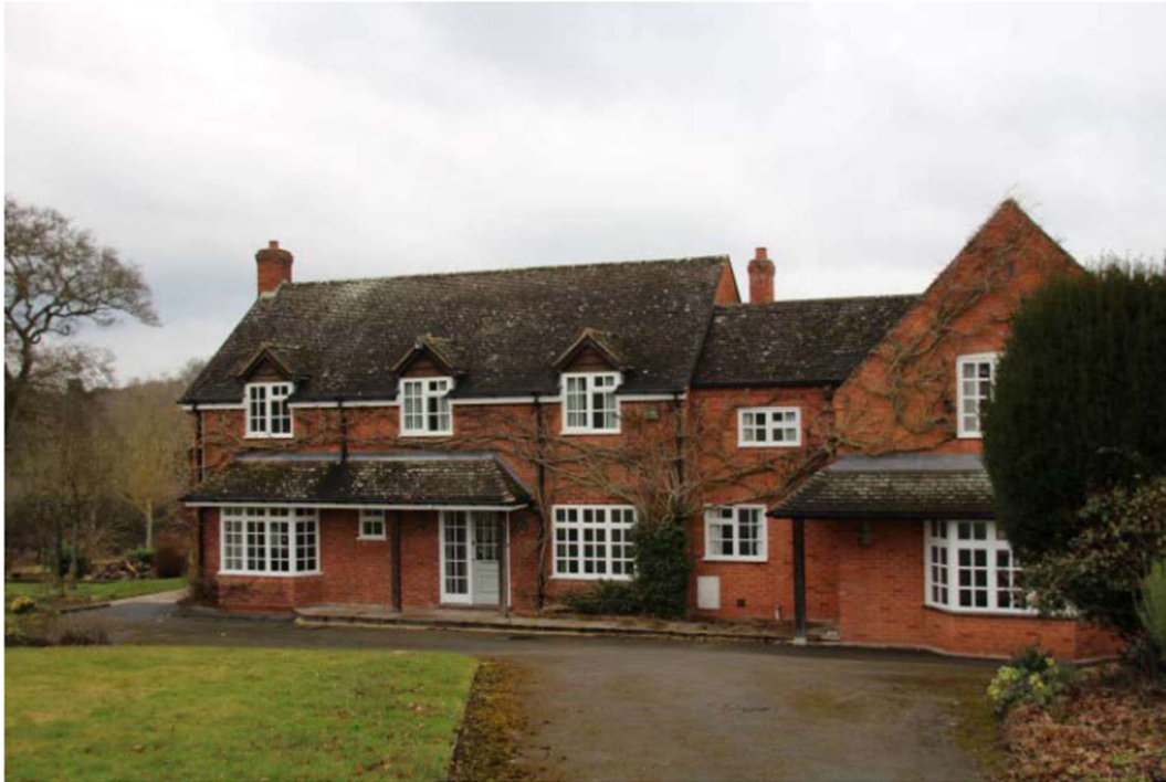
View of existing House from Driveway
