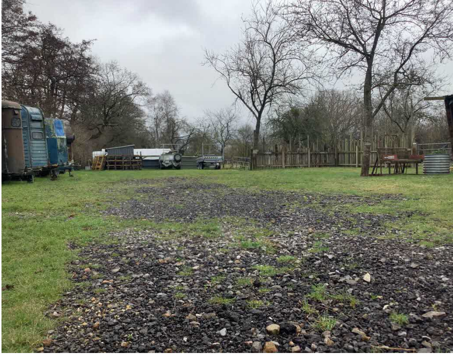
Figure 4. Existing hard-standing area of farmyard to be used as parking area.
