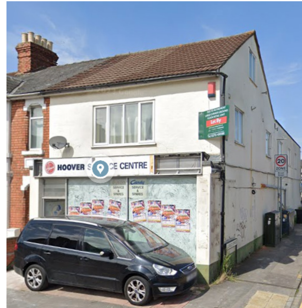
Figure 8 - Existing front elevation of property (Source: Google Maps).
