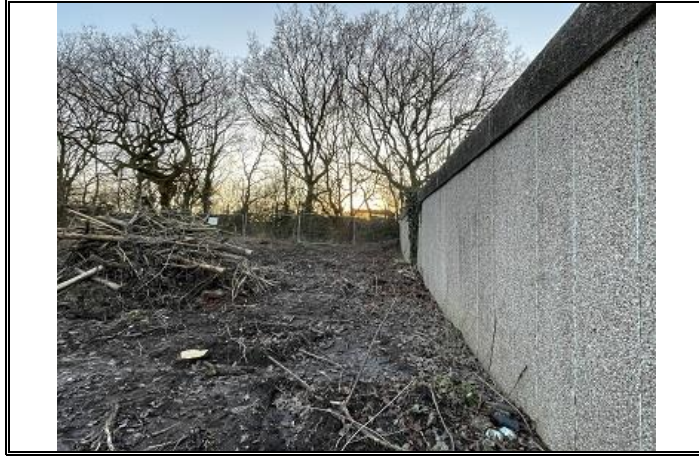
Photo OE/1702/1058/R1/P10 – Rear of southerly garage block.
