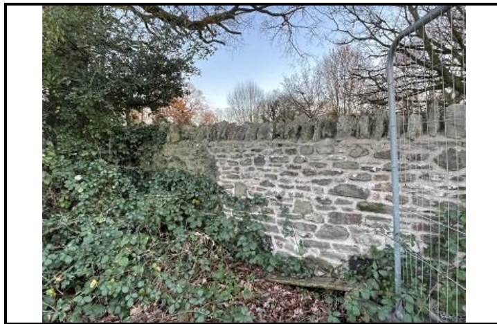
Photo OE/1702/1058/R1/P17 – Southern boundary wall to the site – with churchyard beyond.
