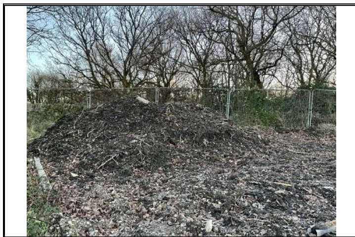
Photo OE/1702/1058/R1/P15 – Southern end of cleared site, with stockpile of vegetation.
