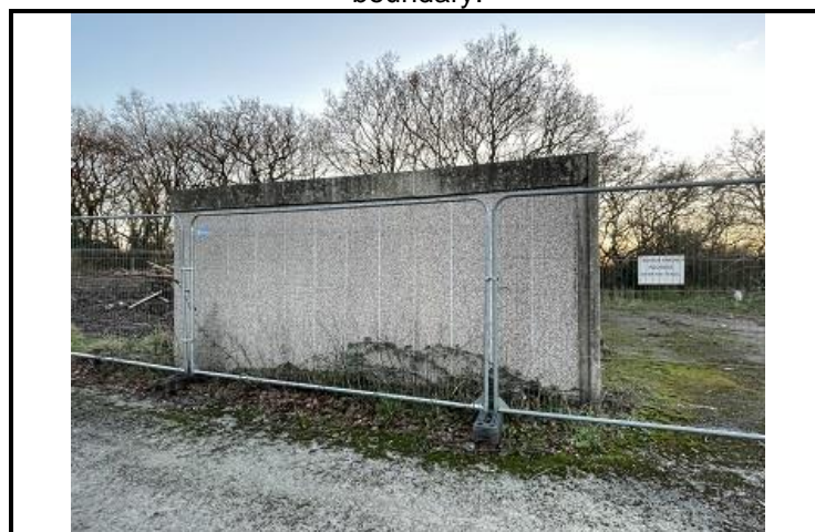
Photo OE/1702/1058/R1/P09 – End of southerly garage block.
