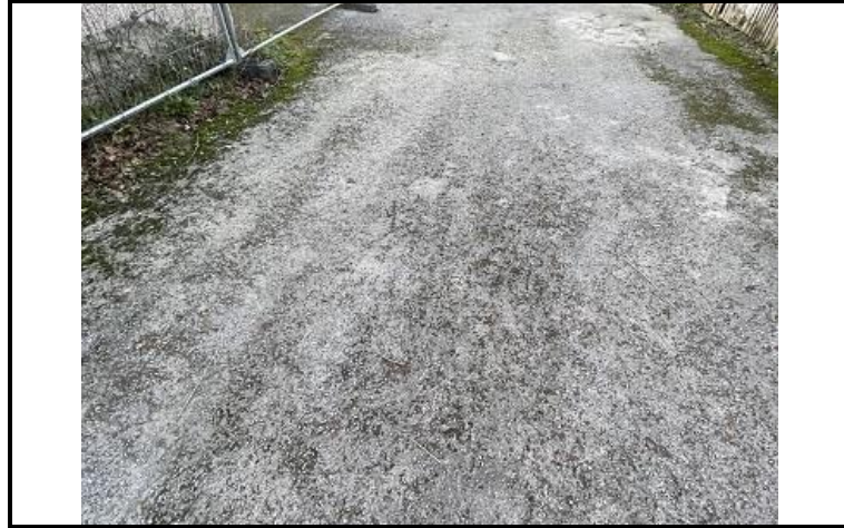
Photo OE/1702/1058/R1/P19 – Existing surfacing to rear access track.
