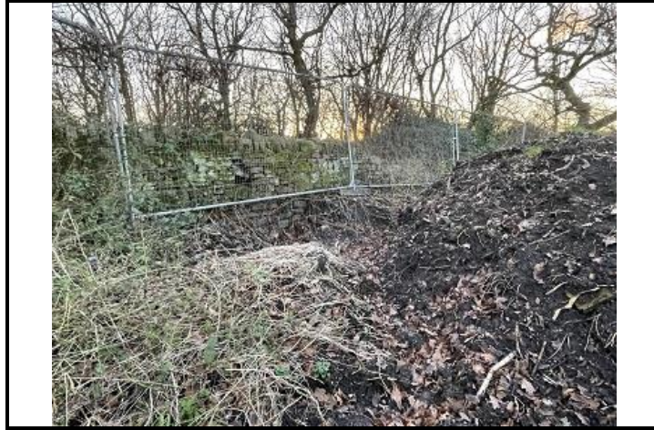
Photo OE/1702/1058/R1/P16 – Southern boundary wall to the site – with churchyard beyond.
