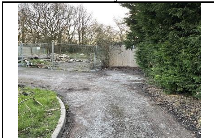
Photo OE/1702/1058/R1/P02 – View towards site form access road – looking east to west.
