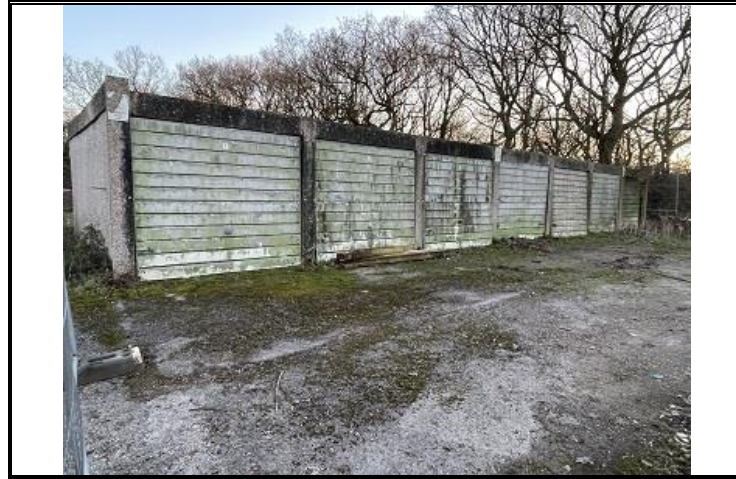
Photo OE/1702/1058/R1/P07 – Southerly row of garages – northern area of the site.
