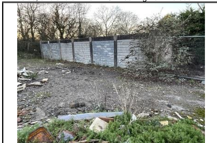
Photo OE/1702/1058/R1/P05 – View of northern garage block.
