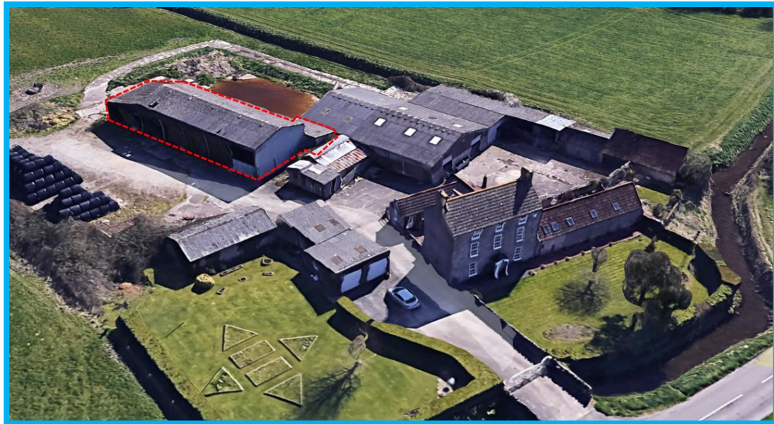
Figure 4 Oblique view of site (looking south) showing general outline of farm building for change of use (Google Earth).
