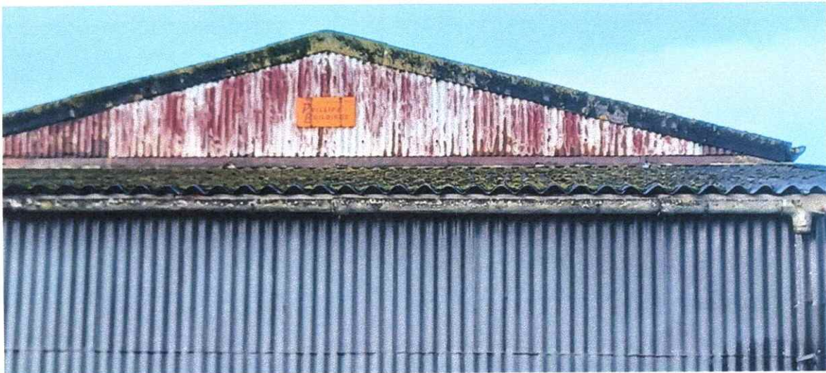
Photograph of east elevation showing lean to and roof structure.
