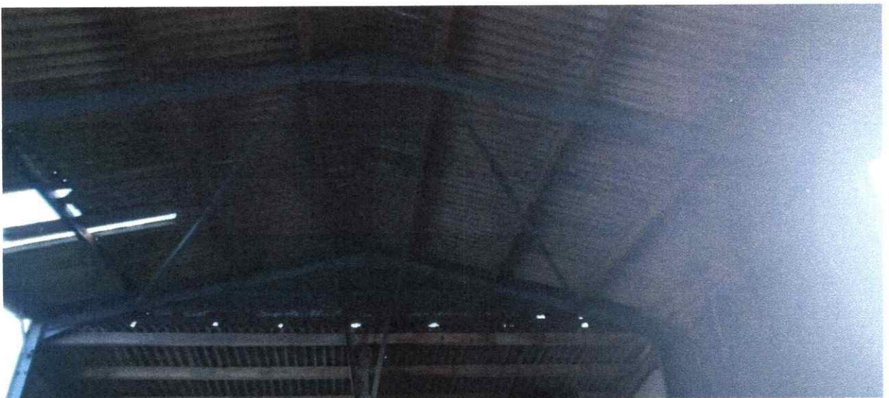
Roof structure with steel members in good condition.
