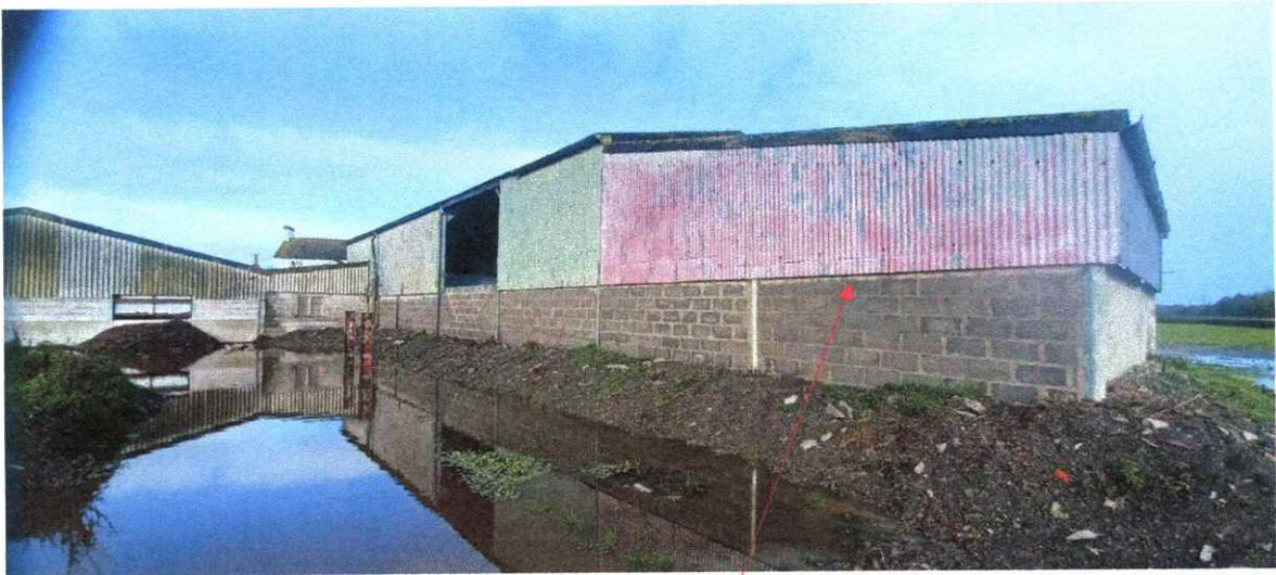
Rear south elevation with lean to on main barn on east elevation
