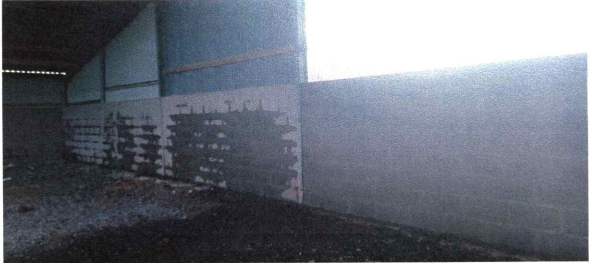
Rear wall to lean to and main barn.
