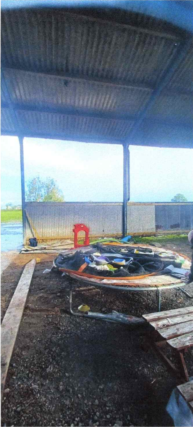
Rafters and column in steel which are in good condition.
