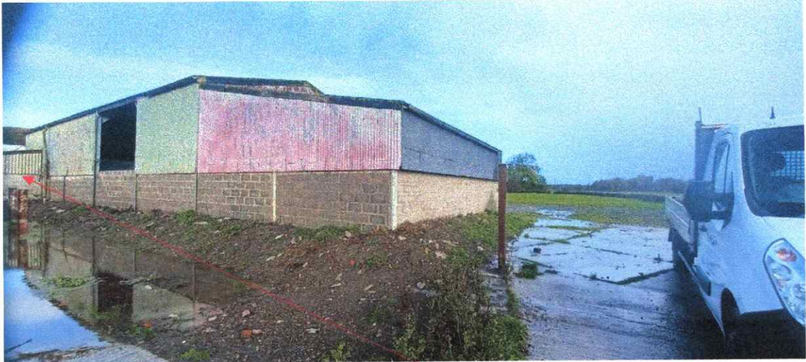
Rear south elevation with lean to link barn in the background
