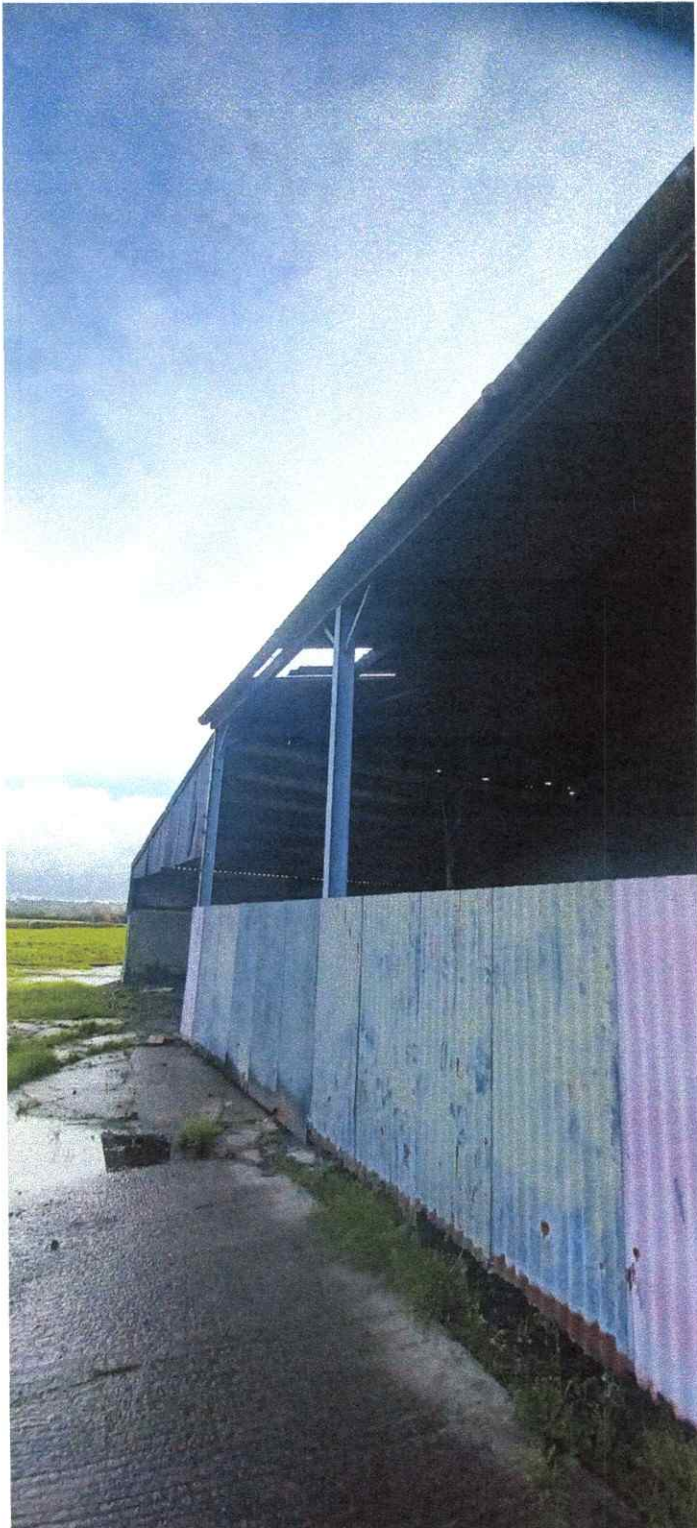
Front north elevation
