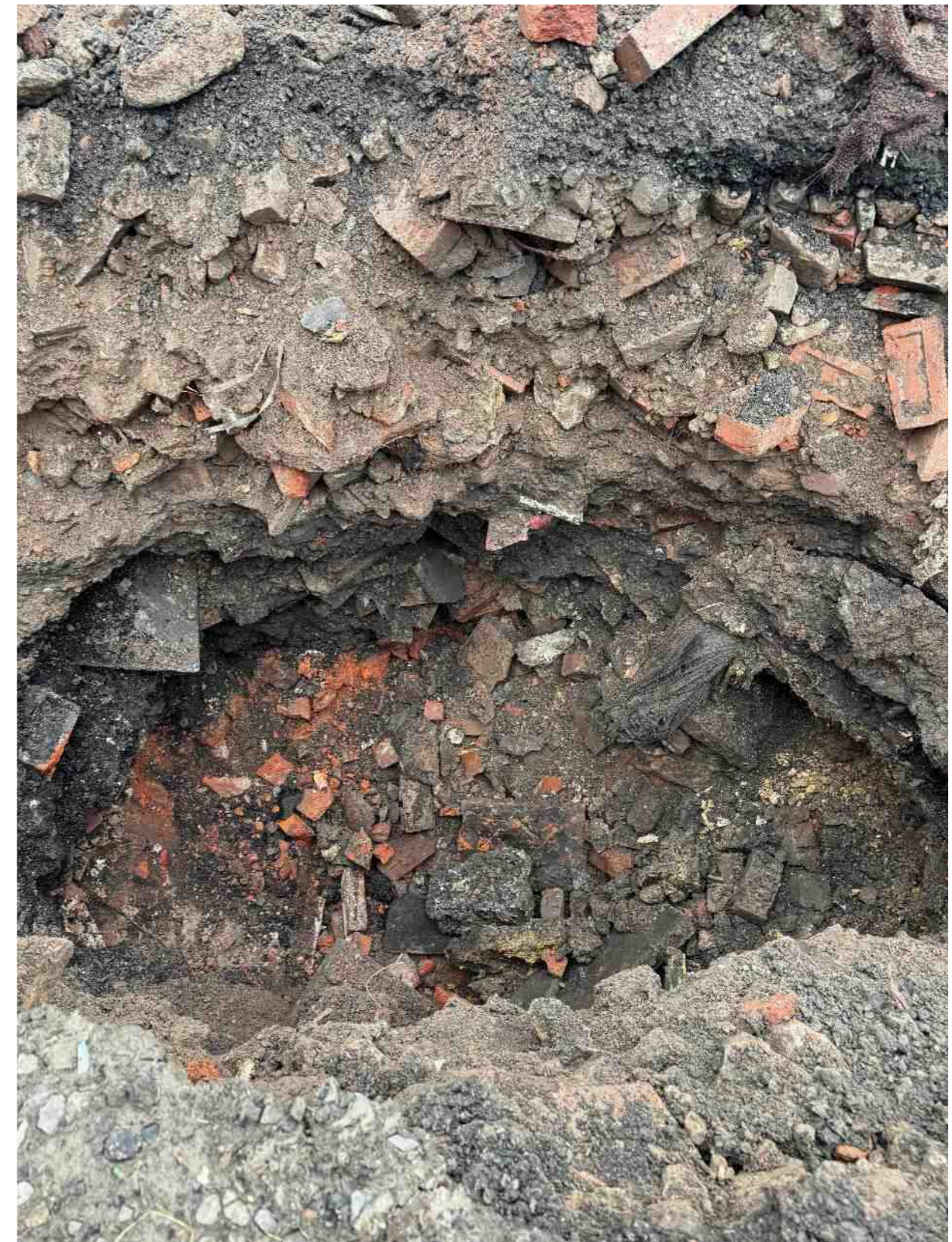
Photograph 1: Trial pit TP101 excavation – 3 m deep, brick fill to base
