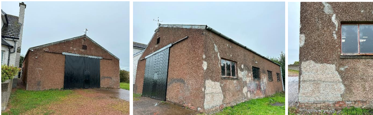
Figure 8: Images of Existing Barn
