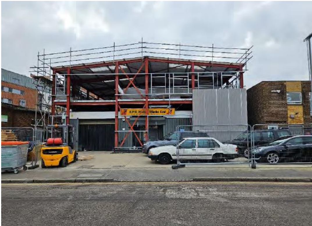
Photographs of the existing premises and ongoing construction works
