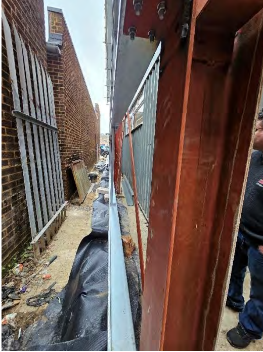
Figure 7: Looking Along the Northwestern boundary
