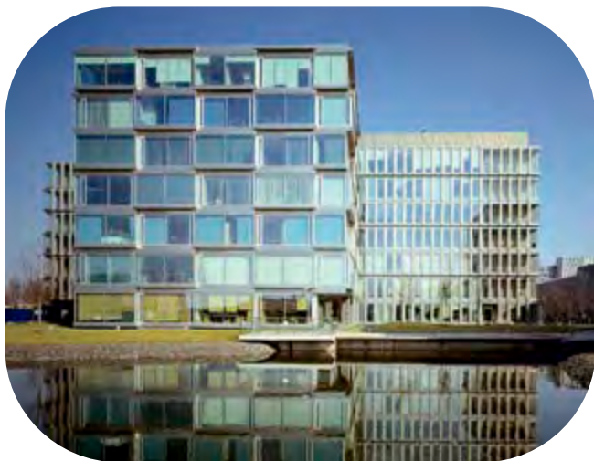
Pilkington Suncool™ 66/33 – Platinum Business Park, Warsaw, Poland
