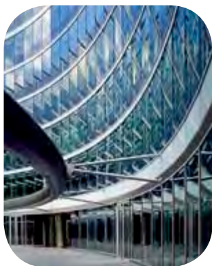
Pilkington Optitherm™ – Metropolitan Building, Warsaw, Poland
