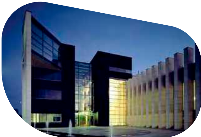
Pilkington Solar-E™ – Comarch SA head office, Cracow, Poland
