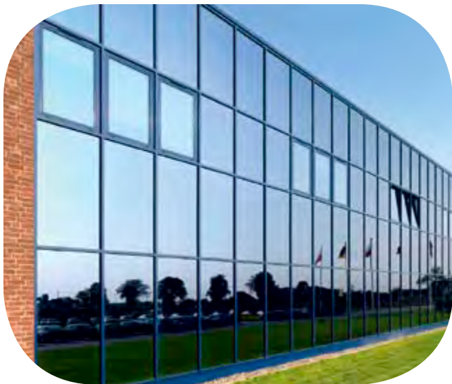
Pilkington Spandrel Glass Coated E130 – Vorwerk Autotec Polska head office, Brodnica, Poland
