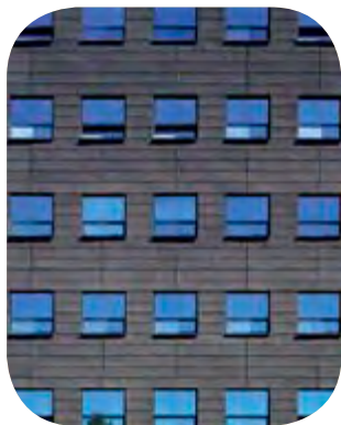
Pilkington Suncool™ 50/25 – Aeropark Business Center (building A), Warsaw, Poland
