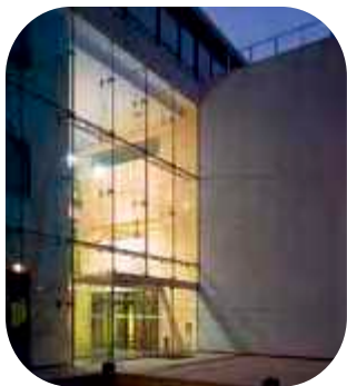
Pilkington Planar ™ – Hector Training Centre, Warsaw, Poland
