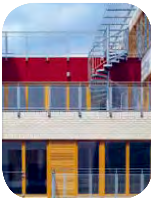
Pilkington Optilam ™ 9,5 – Eko-Park housing estate, Warsaw, Poland
