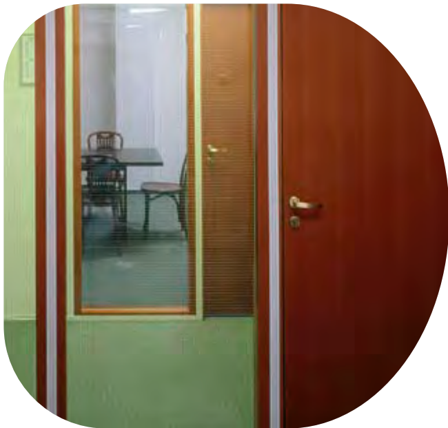
Pilkington Pyroshield™ 2 – Agora`s printing house, Warsaw, Poland
