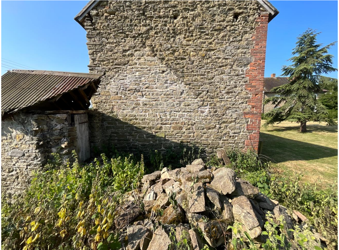
Plate 3 - Outline of former cattle shed visible on stable range farm building and old privy to the left, which will be retained.
