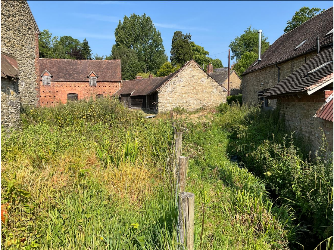
Plate 2 – Former agricultural buildings - neighbouring listed building 'The Chains and outbuilding to south west' to the right of the stream.
