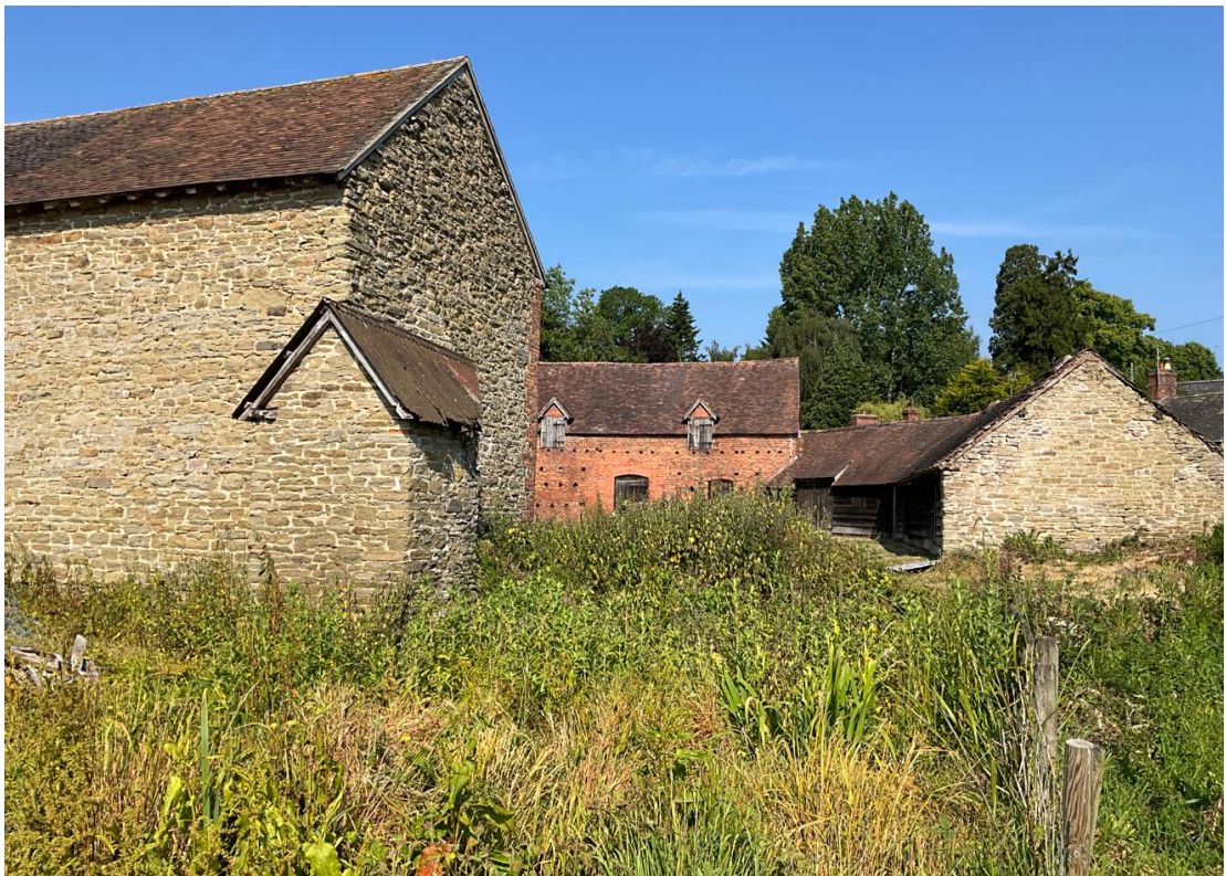
Plate 1 – The former agricultural buildings at Munslow Farmhouse. The red brick barn in the background, remaining enclosed portion of the cattle shed to the right of the photograph and stable range with granary above to the left of the photograph, and stream to the right of the boundary posts. The remains of the privy can also be seen attached to the corner of the stable range.
