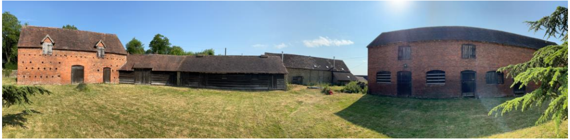
Plate 5 - Panoramic shot of the range of outbuildings and grade II Listed 'The Chains' to the rear.
