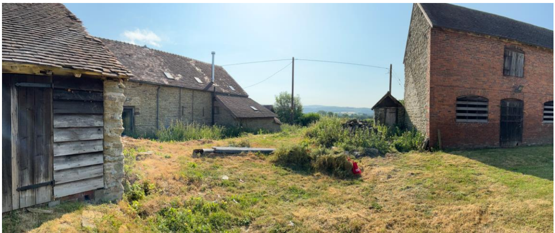
Plate 4 - Space in between weatherboarded cattle shed and brick faced stable and granary building where previously demolished open bays of the cow shed once stood.
