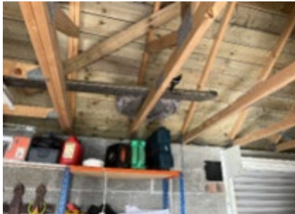
Picture 5 – Cable to run along the top
