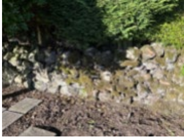
Picture 3 – Cable to run against wall.
