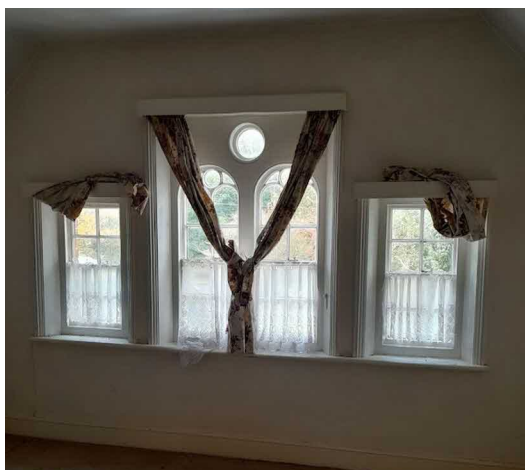
First floor front window
