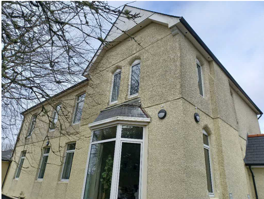
Figure 7: View of south elevation of two-storey section of Meadowbrook House.
