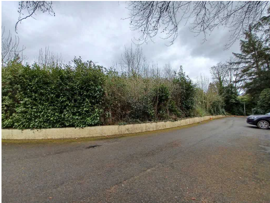
Figure 3: View of wall, with introduced shrubs and scattered trees beyond.
