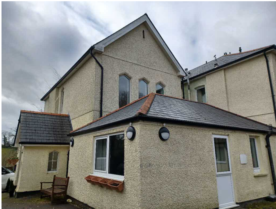
Figure 4: View of north elevation of two-storey section of Meadowbrook House.
