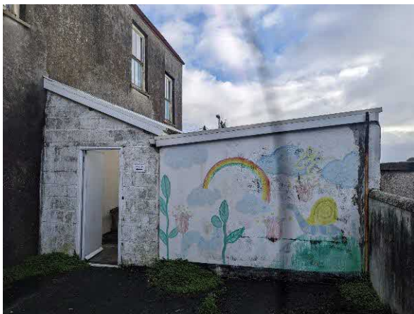
Photo 4. Showing the toilet block and covered courtyard from the west
