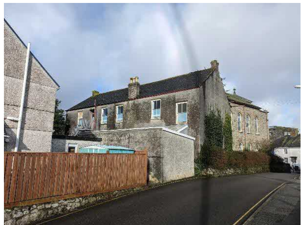
Photo 2. Showing the School rooms from the south
