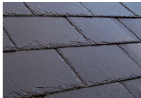
Reclaimed natural slate roof with lead valleys
