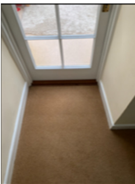
Door to existing conservatory
