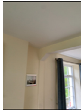
Original wall to be reinstated
