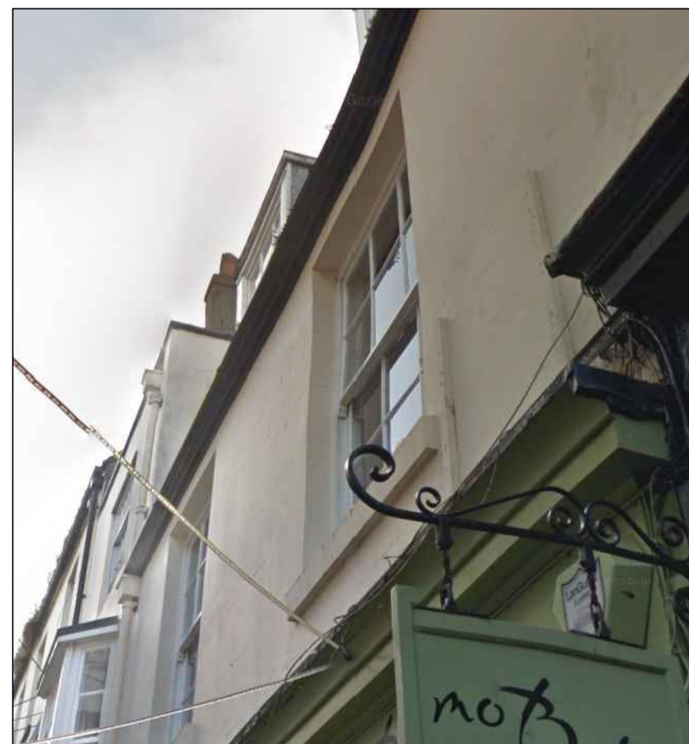
First Floor Typical Sash Window (External) facing Union Street
