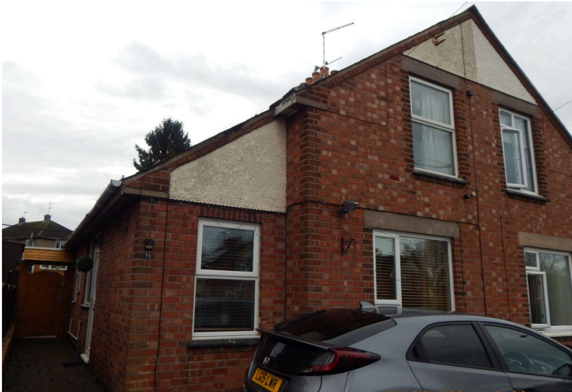
Image 1 – Front North facing elevation of the property
