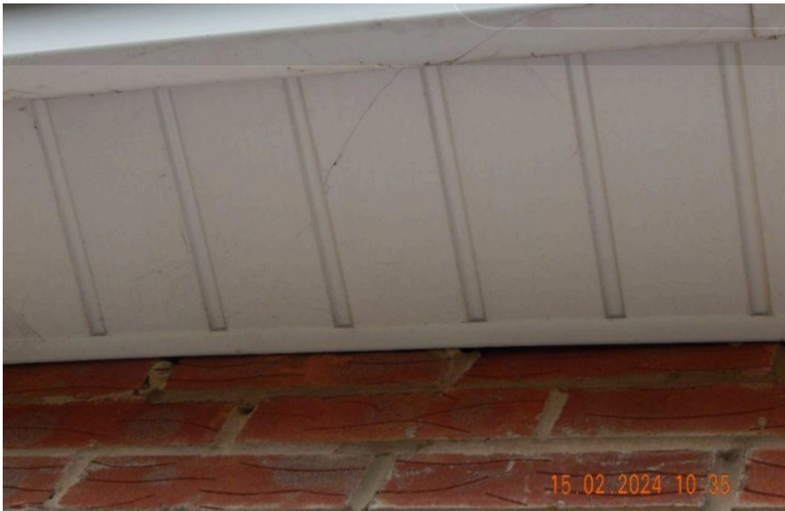
Image 5 – Close view of the eaves coverings to demonstrate example of condition
