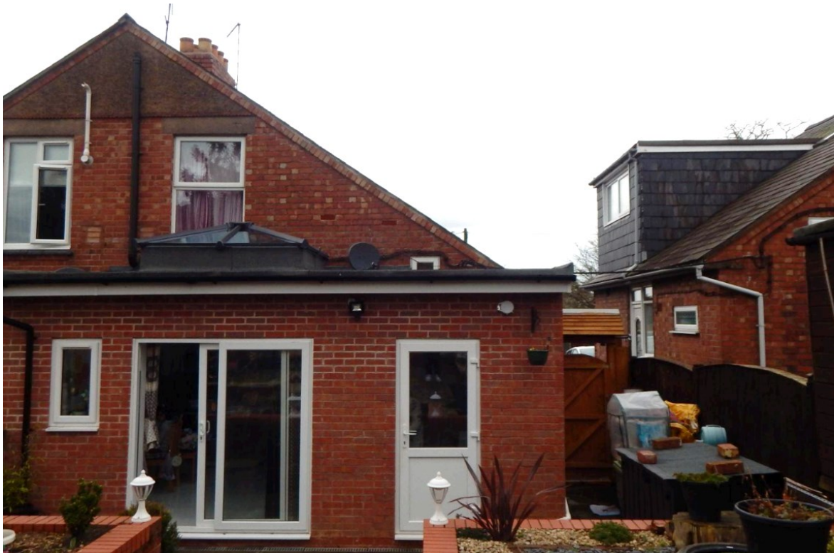
Image 2 – Rear South facing elevation of the property
