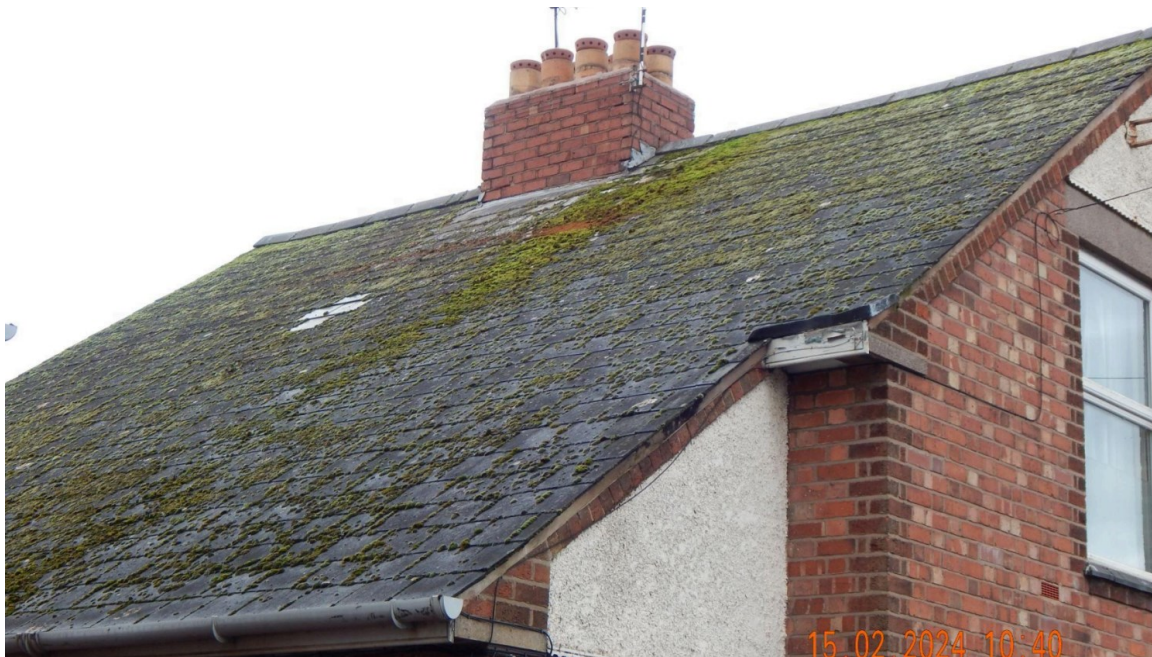
Image 3 – East facing elevation/roof coverings of the structure
