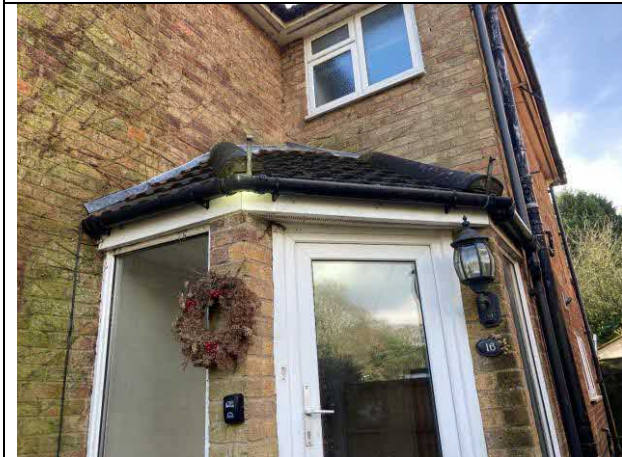
Photo 3 Porch north elevation
