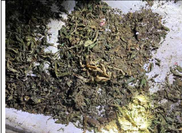
Photo 5 Old plant growth loft floor
