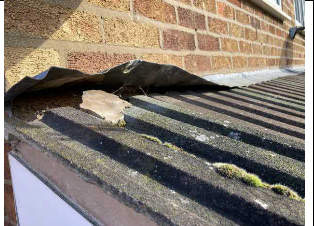
Photo 6 PRF rear single storey section
