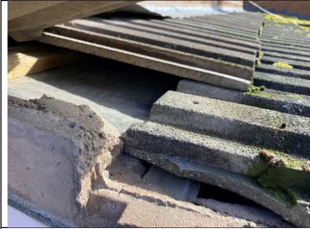
Photo 7 PRFs single storey section
