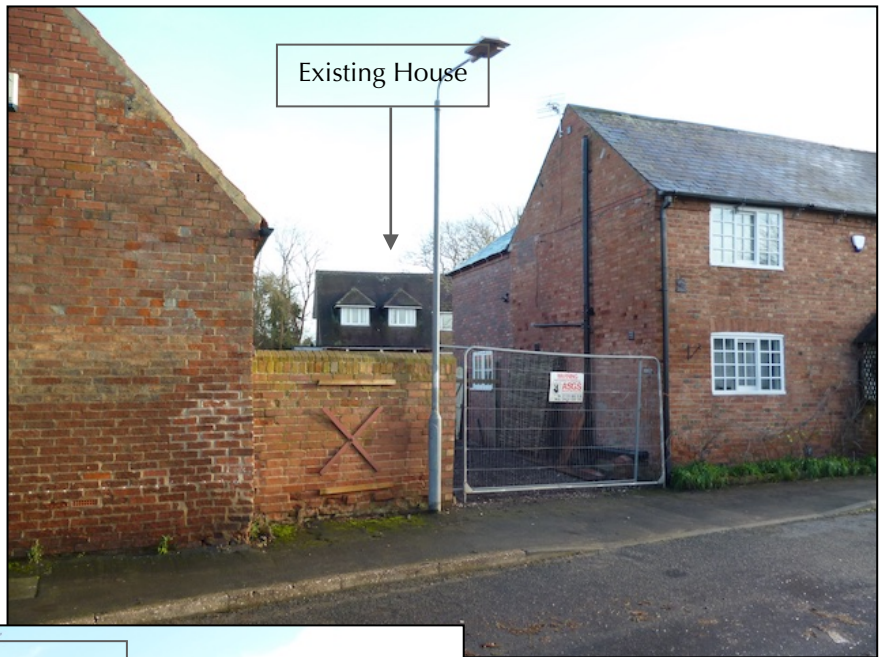
Photo 6: General view looking between nos 12 & 14, Moor Lane with a glimpsed view of the existing house in the background
