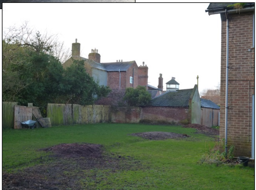
Photo 11: View of the rear elevation of the Old Vicarage and the range of single storey outbuildings
