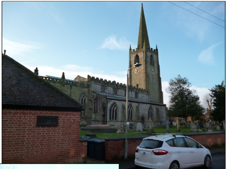
Photo 12: View of the St Mary's Church from Church Street
