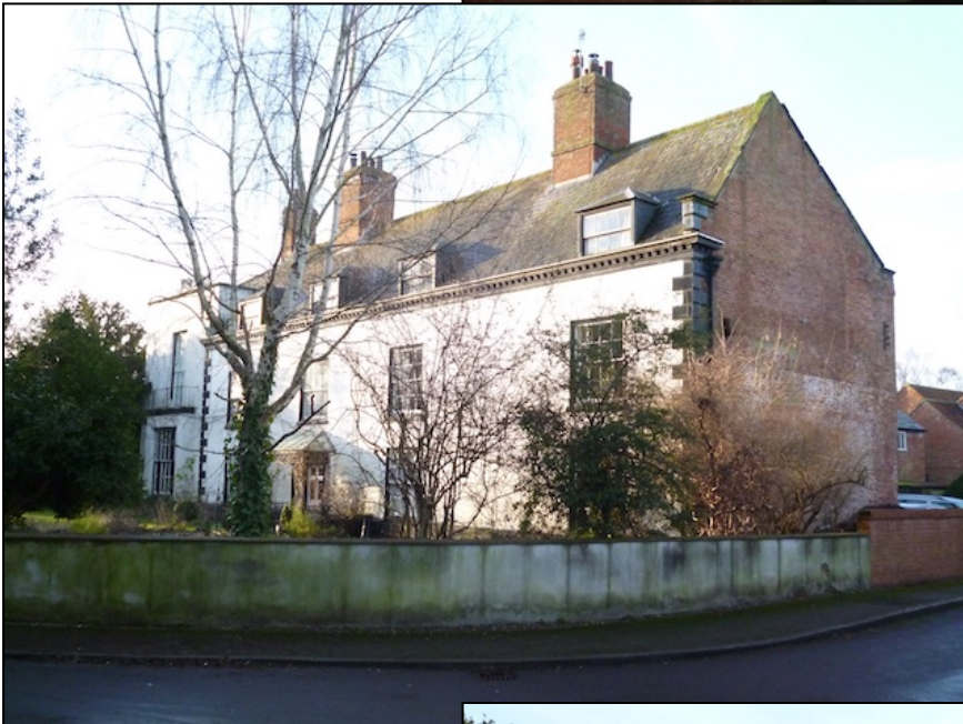
Photo 13: View of the front elevation of The Grange from Moor Lane
