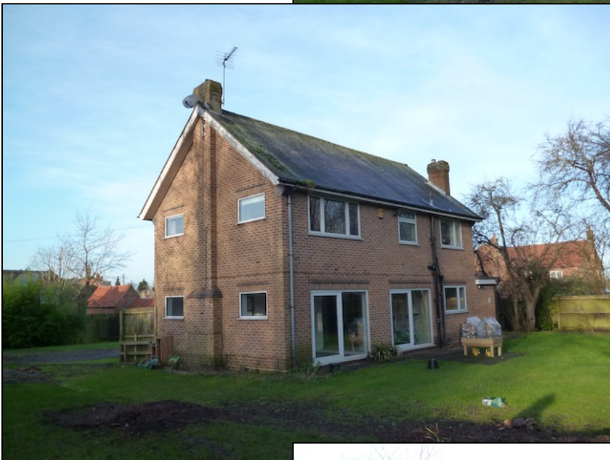
Photo 2: General view of the rear elevation of the existing property
