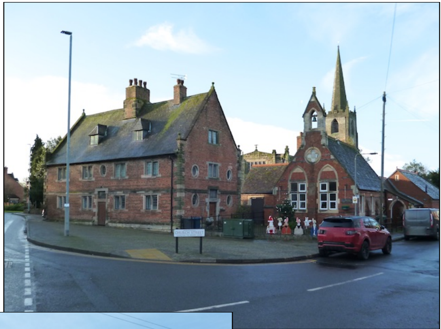
Photo 15: View of the Parish Rooms on Church Street and the former school on Loughborough Road
