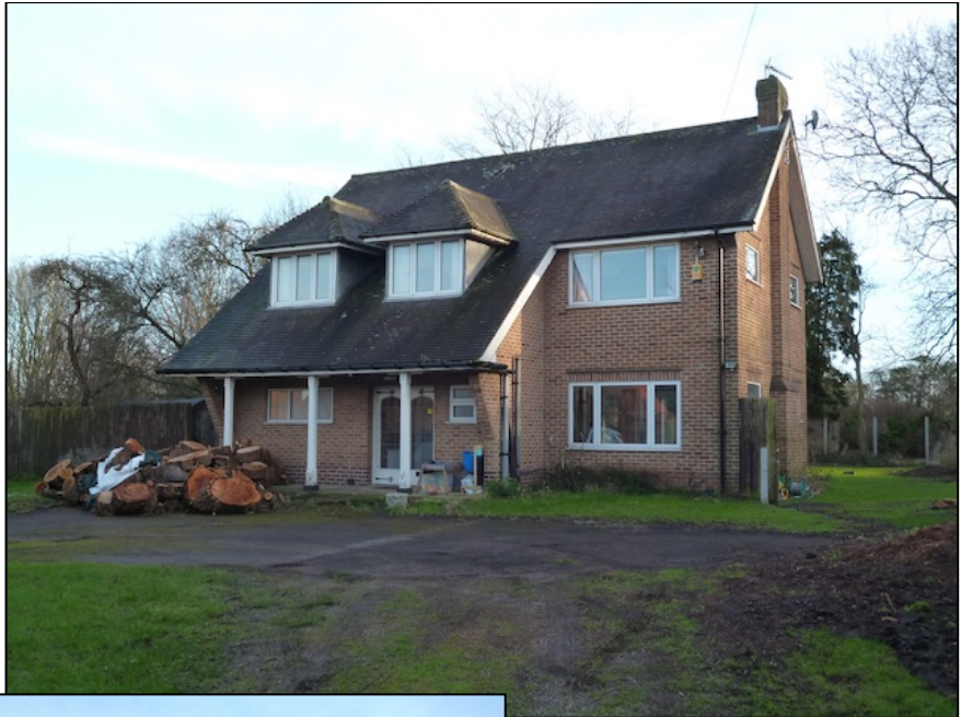
Photo 1: General view of the front elevation of the existing property
