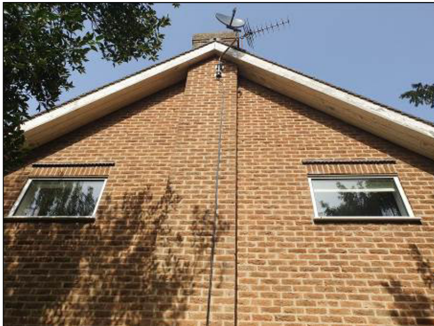
Photograph 3 - Southern aspect of building
