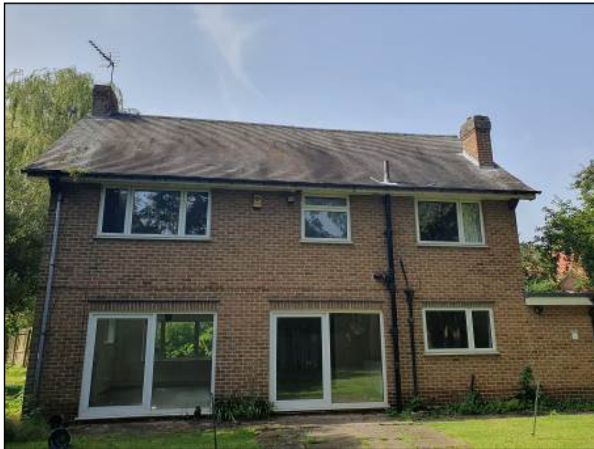
Photograph 2 - Eastern aspect of building
