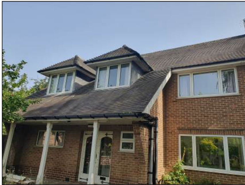
Photograph 4 - Western aspect of building
