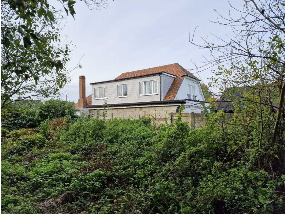
Photo 11 – View of No. 13 looking south-west from within site.
