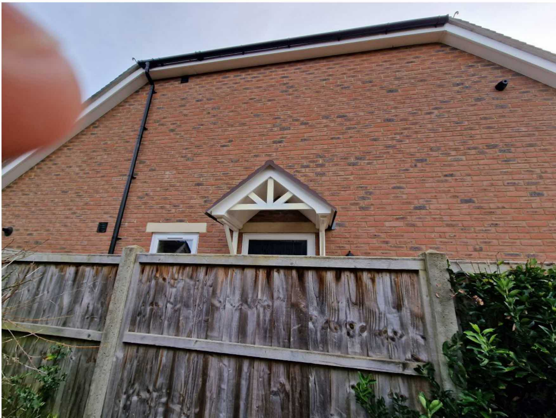
Photo 10 – View of west flank of No. 17a from within site.
