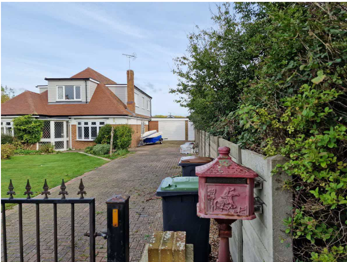
Photo 8 – View looking north from New Cut of No. 13 with western site boundary to right.
