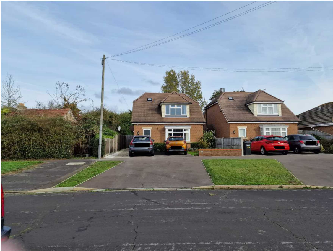
Photo 3 – View looking north of Nos. 17a & 17b with existing cottage (No.15) just visible to left.
