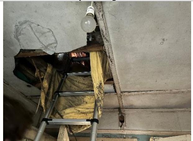
The bungalow does not have a loft hatch but the loft void can be accessed from the broken part of the ceiling
