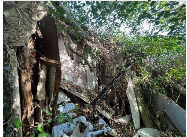
Western side of the southern aspect of the surveyed bungalow
