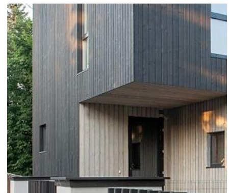
Fig 6. Examples of proposed materials, standing seam roof, dark charred vertical timber cladding
