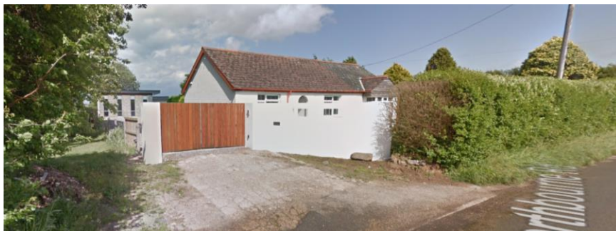
Fig 8. Existing street scene – tall boundary hedgerow screens house from road
