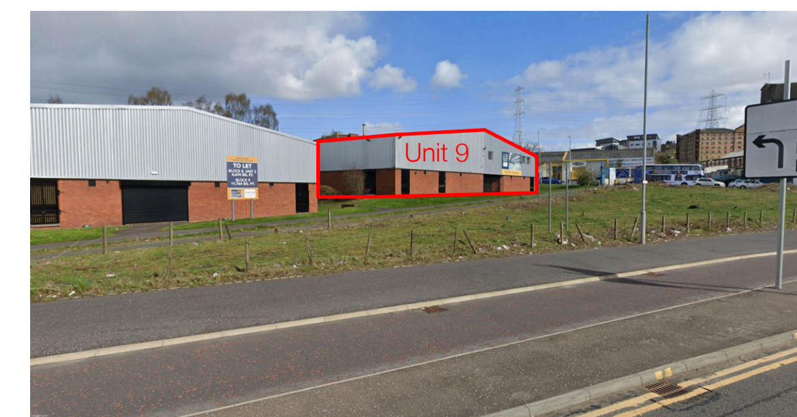
View from Garscube Road
