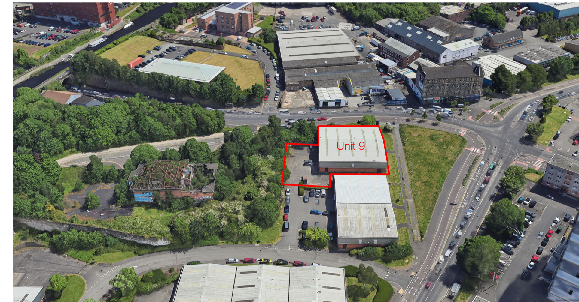
View from West, towards service yard
