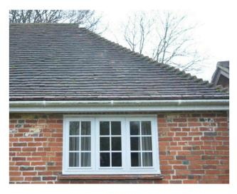
The window shown above is to the far right of the property. This window will be removed along with brickwork below to form a new opening for patio doors.
