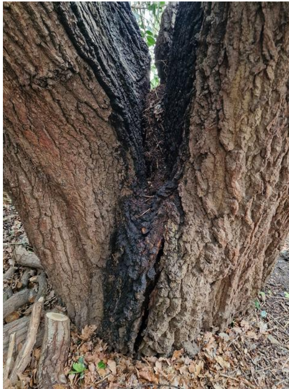
Image 13 T226 an oak tree with a separation sheer crack.
