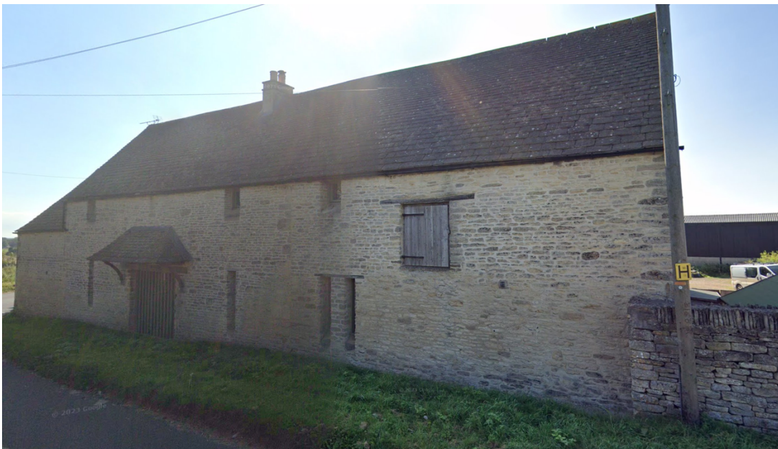
Photo: Roadside view of The Barn
