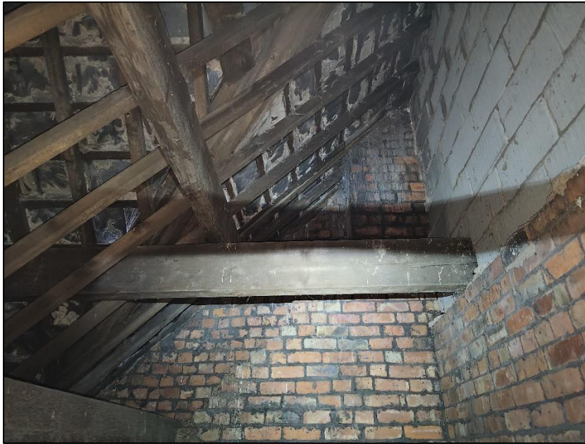
Photograph 10 showing one of the roof voids.
