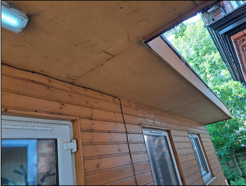
Photograph 12 showing the timber-clad annexe.
