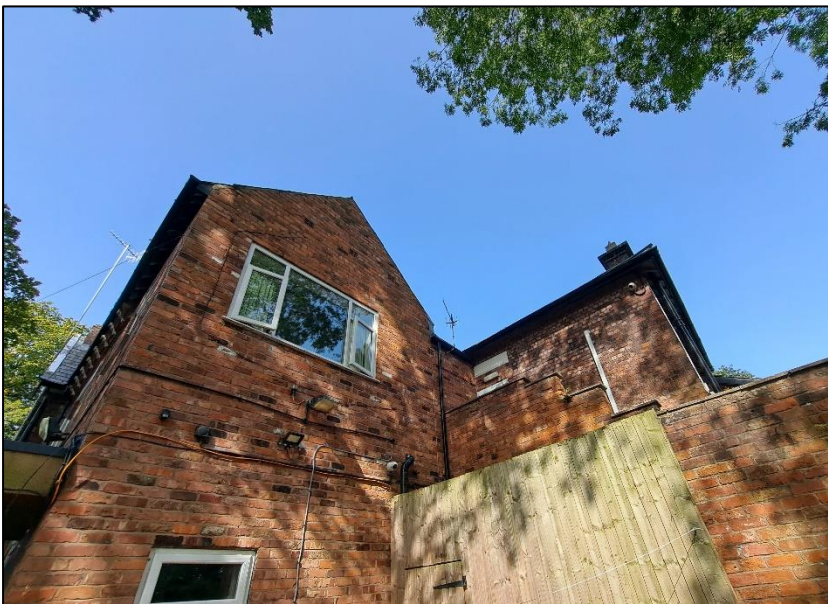
Photograph 5 showing the rear elevation.
