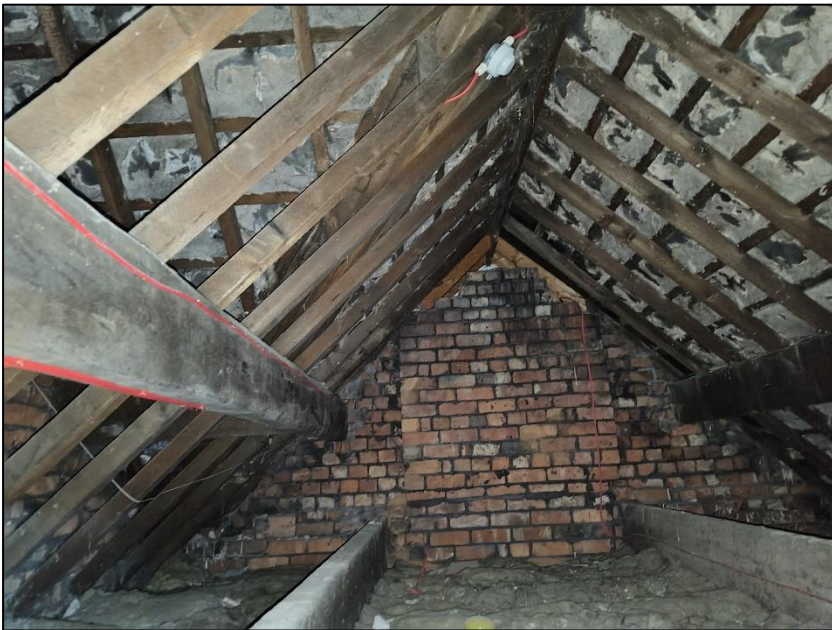
Photograph 9 showing one of the roof voids.
