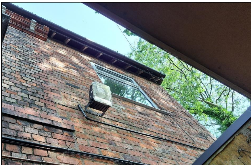
Photograph 7 showing the exposed roof joists.
