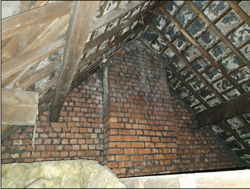
Photograph 8 showing one of the roof voids.
