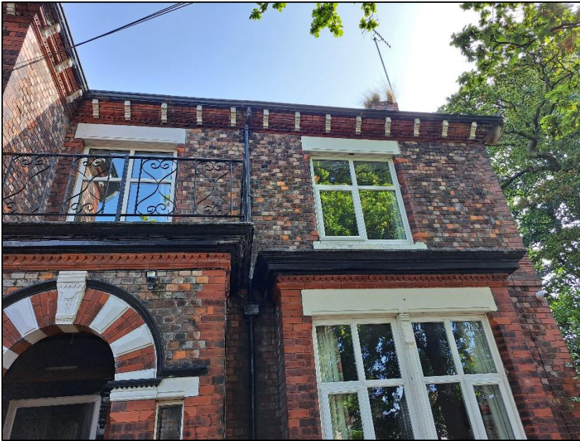
Photograph 4 showing the exterior of the building.
