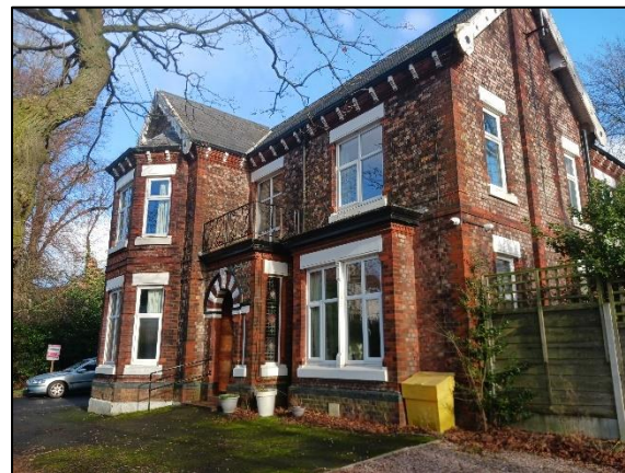
Figure 4: View of front (west) and side (south elevations).
