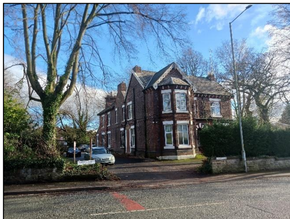
Figure 3: View of 34 Sandy Lane from Sandy Lane.
