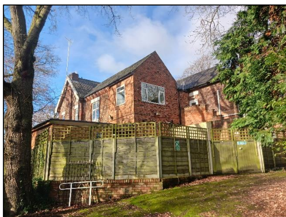
Figure 5: Partial view of the rear (east) and side (south) elevations
