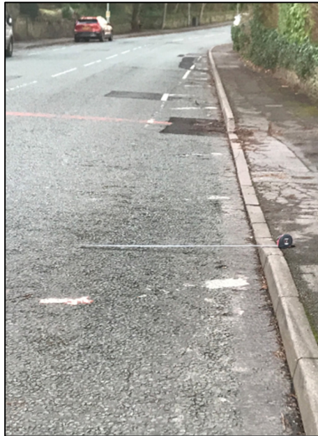
Plate HTN5 - Extent of hatching to front of application site (circa 1.1m - 1.2m) and demonstration of improved visibility achievable.
