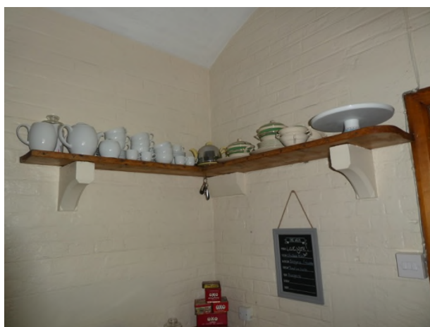
Figure 31: Stone brackets for shelves on the south-west side of the kitchen
