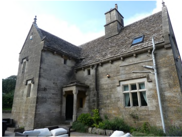
Figure 14: South elevation viewed from the south-east
