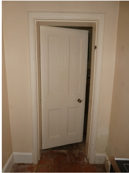
Figure 20: 4-panelled door to the dining room
