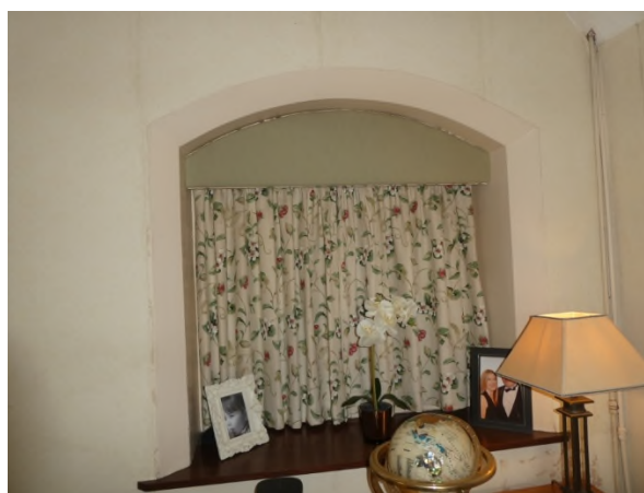
Figure 29: Detail of a blocked window on the north side of the sitting room
