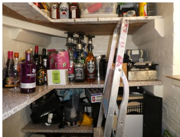
Figure 37: Stone brackets for shelves in the under stairs cupboard
