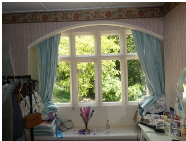
Figure 41: Mullion and transom window on the east side of Bedroom 1
