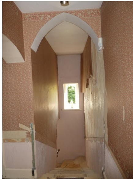
Figure 56: 2-pointed arch at the top of the stairs
