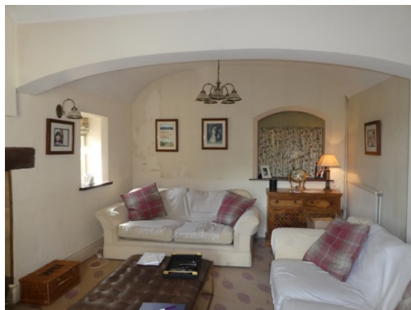
Figure 28: North side of the sitting room with the segmental arch defining the position of an original wall
