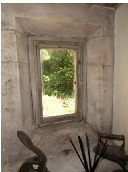
Figure 53: Pivotal window on the east side of the cupboard
