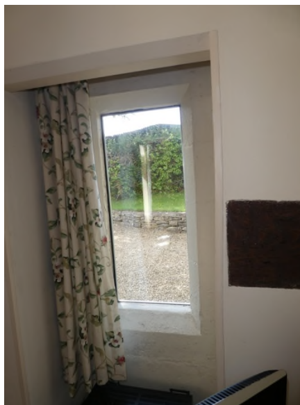
Figure 26: window with chamfered stone frame to the left of the fireplace
