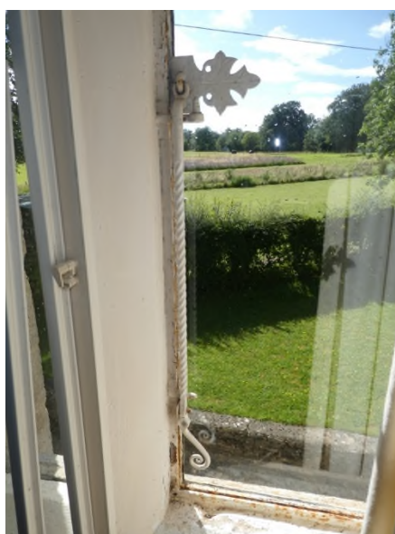
Figure 49: Detail of the window fittings in bedroom 4
