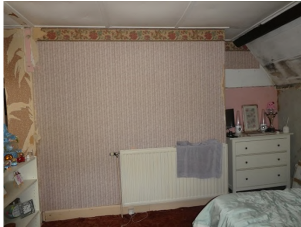
Figure 40: Chimney breast in Bedroom 1
