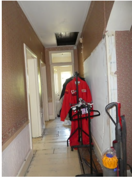
Figure 55: Landing leading to bedrooms 3 and 4
