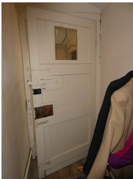
Figure 39: Original back door with a later glazed panel
