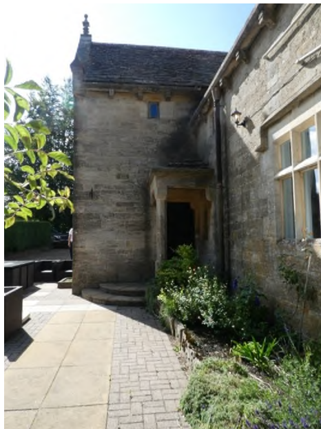
Figure 17: East elevation of the stair turret and porch
