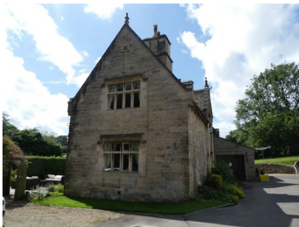
Figure 18: East elevation of the main part of the house
