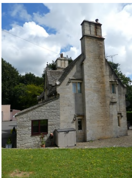
Figure 19: West elevation of The Lodge House
