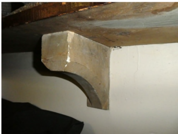
Figure 52: Stone bracket for wooden shelves in the cupboard
