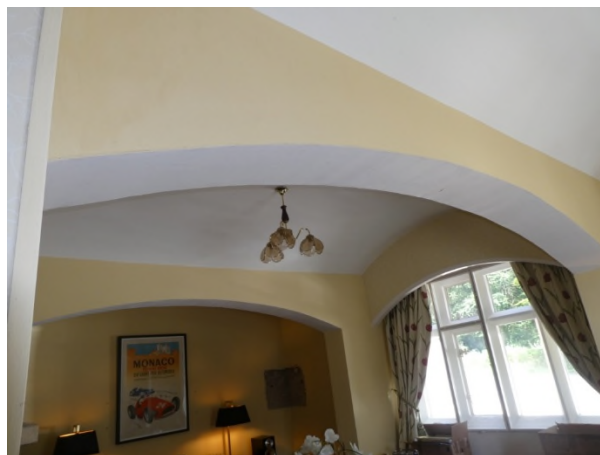
Figure 21: Vaulted ceiling and transvers arches in the dining room
