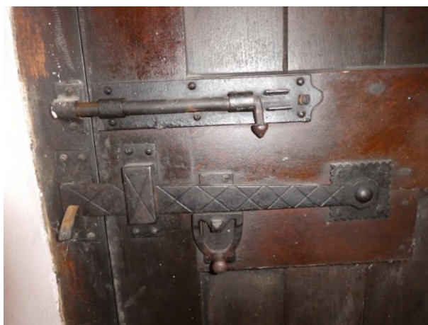
Figure 34: Original latch on the front door
