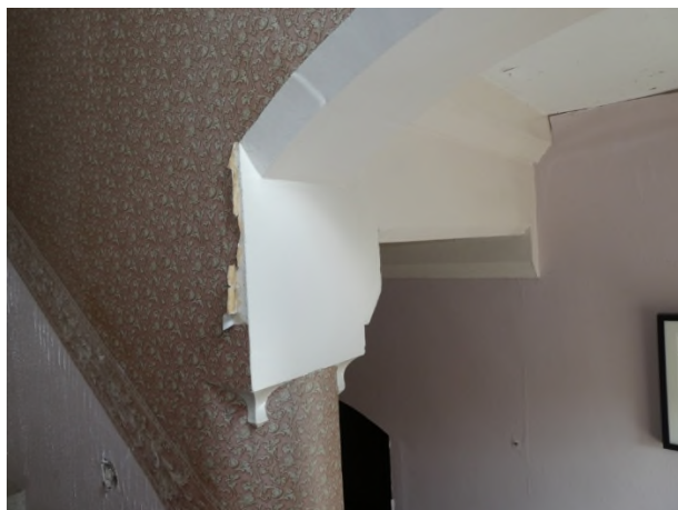
Figure 57: Chamfered segmental arch and pendant details
