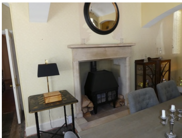
Figure 22: Stone fire surround with chamfer and stop details
