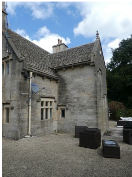
Figure 15: South elevation viewed from the south-west
