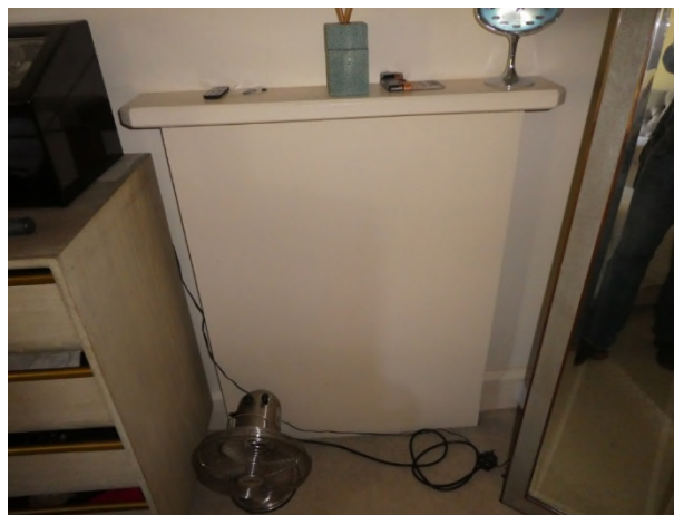
Figure 46: Blocked fireplace on the east side of bedroom 2
