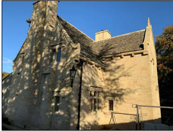
Photo 3 South west elevation
