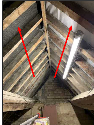
Photo 10 Internal loft main house
