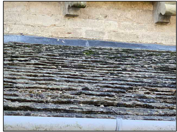
Photo 8 Tiles on extension
