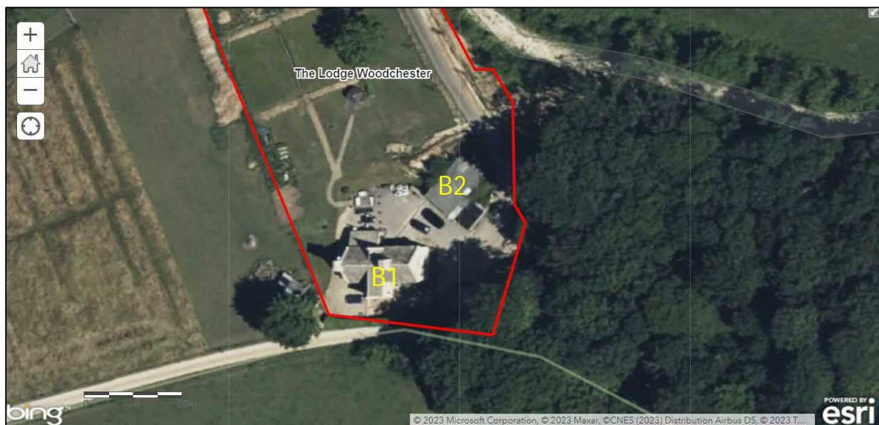
Figure 5 Structures on site
