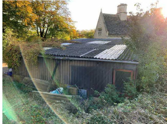
Photo 13 Rear north elevation of garage
