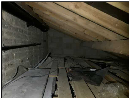
Photo 11 Loft void above extension
