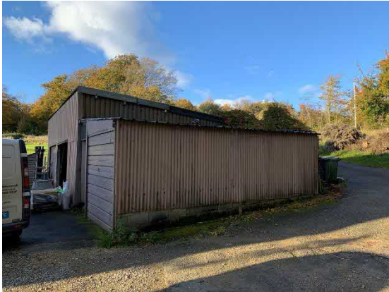
Photo 12 South east elevation of garage
