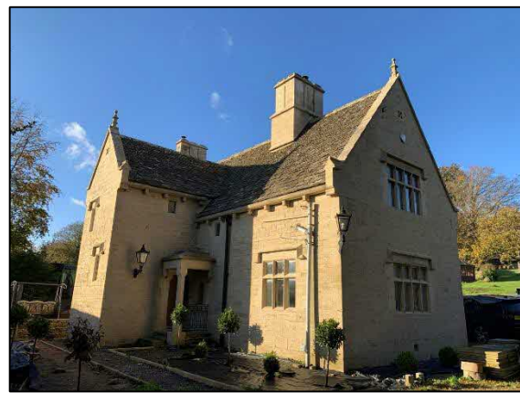
Photo 2 South east elevation
