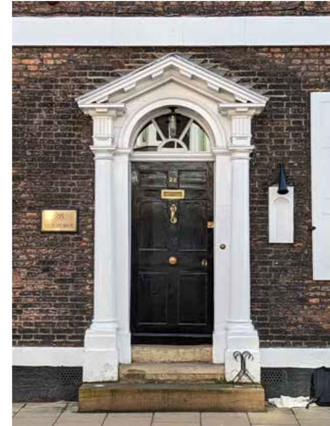
Overall view of doorway
