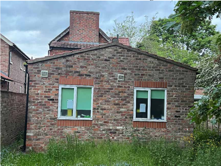
Plate 4 – Old School, south gables.
