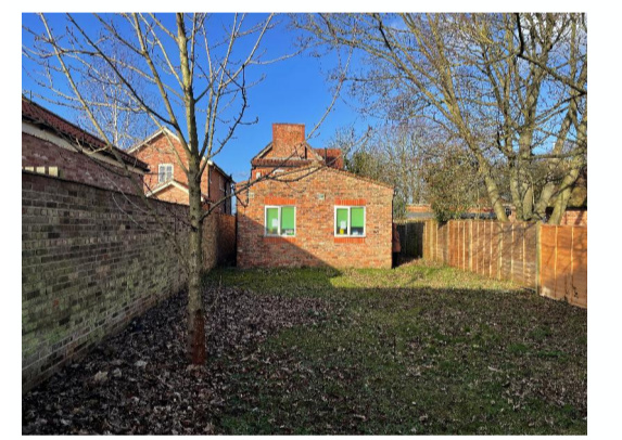
46 Church Lane - Rear View
